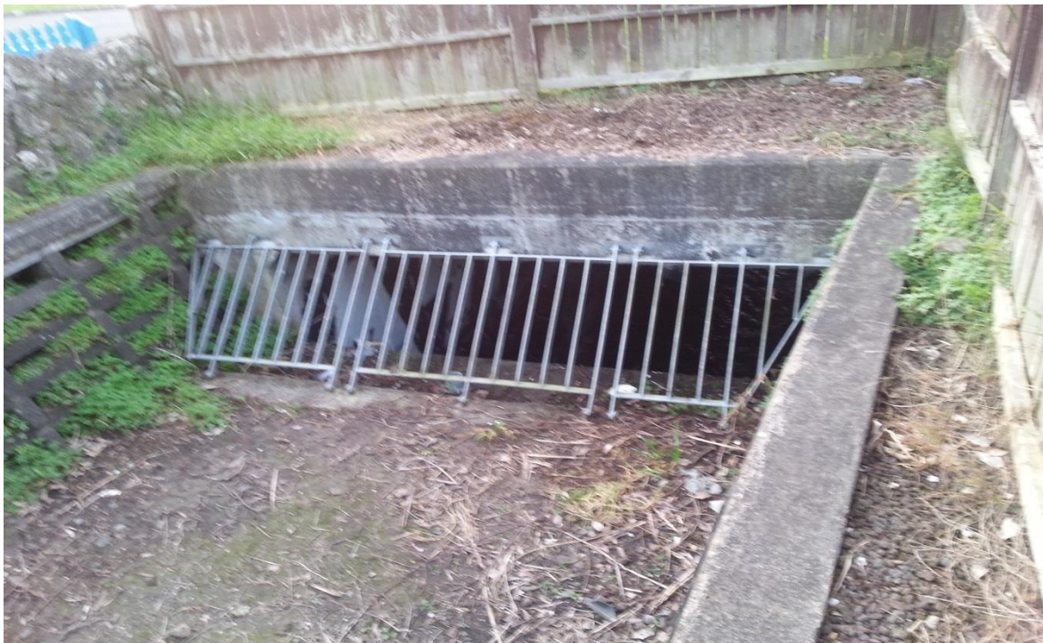
Figure 3-2 Culvert Inlet under Linwood Avenue
