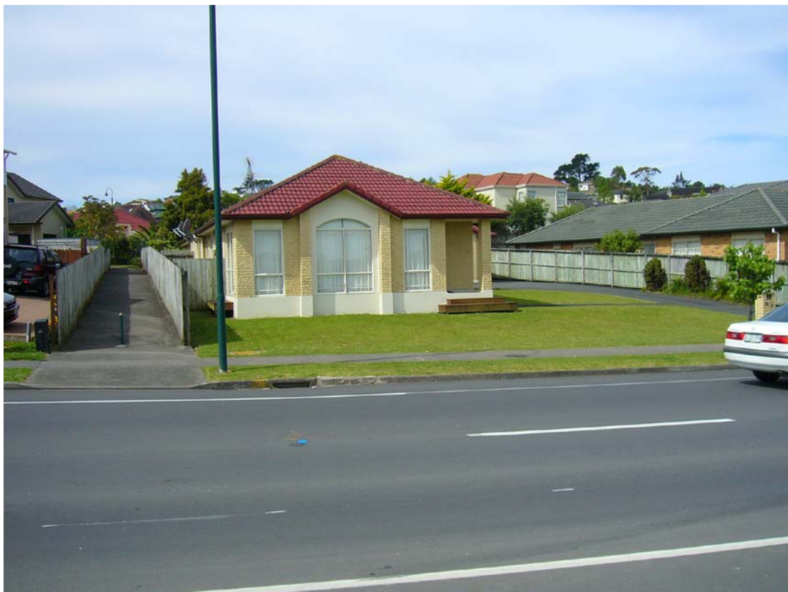
Photo 5.15 30 Hugh Green Drive within the overland flow path floodplain
