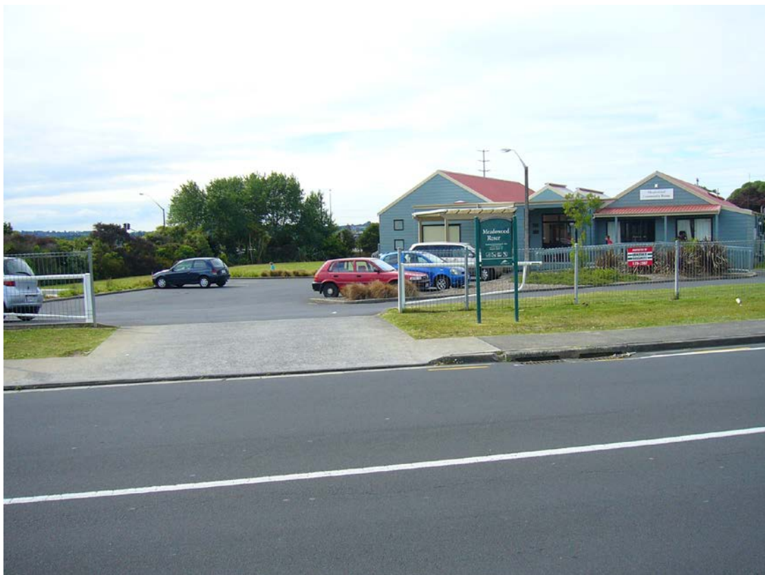
Photo 5.13 55 Meadowood Drive within the overland flow path floodplain
