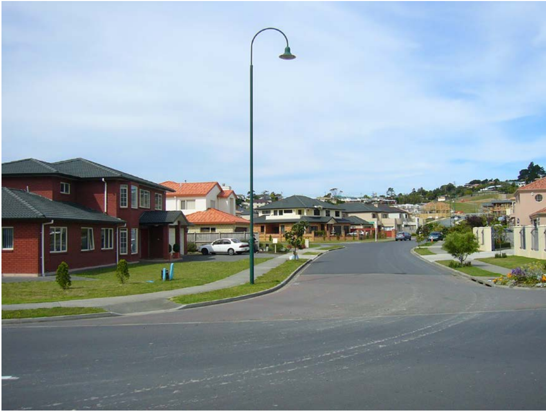
Photo 5.16 122 Hugh Green Drive within the overland flow path floodplain
