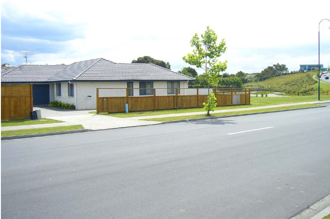
Photo 5.17 101 Hugh Green Drive within the overland flow path floodplain
