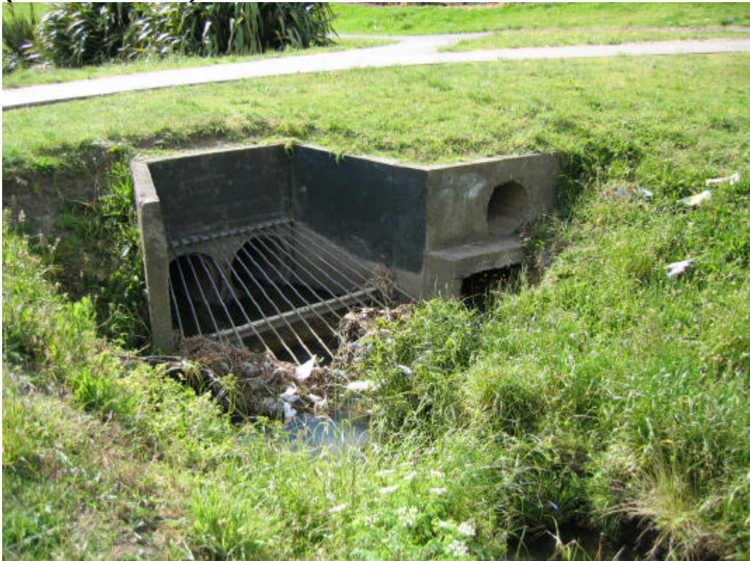
Figure J4: Culvert Behind 42 Maybury Avenue (Maybury Reserve) (December 2003)
