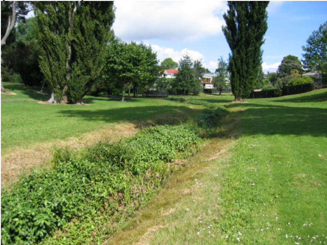
Figure J15: View Upstream of 47 Dunkirk Road (Johnson Reserve) (December 2003)
