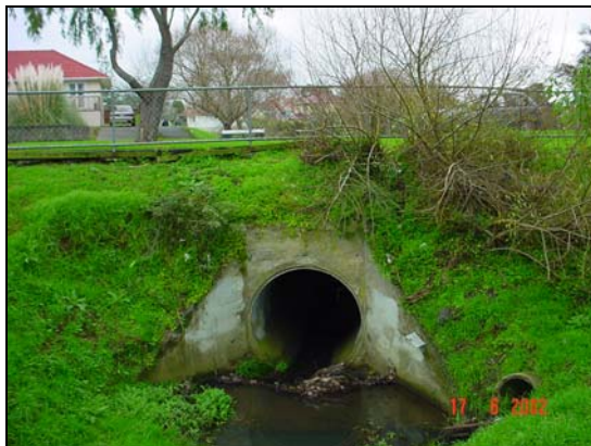
Figure 2.2 Upstream End – 17 June 2002
