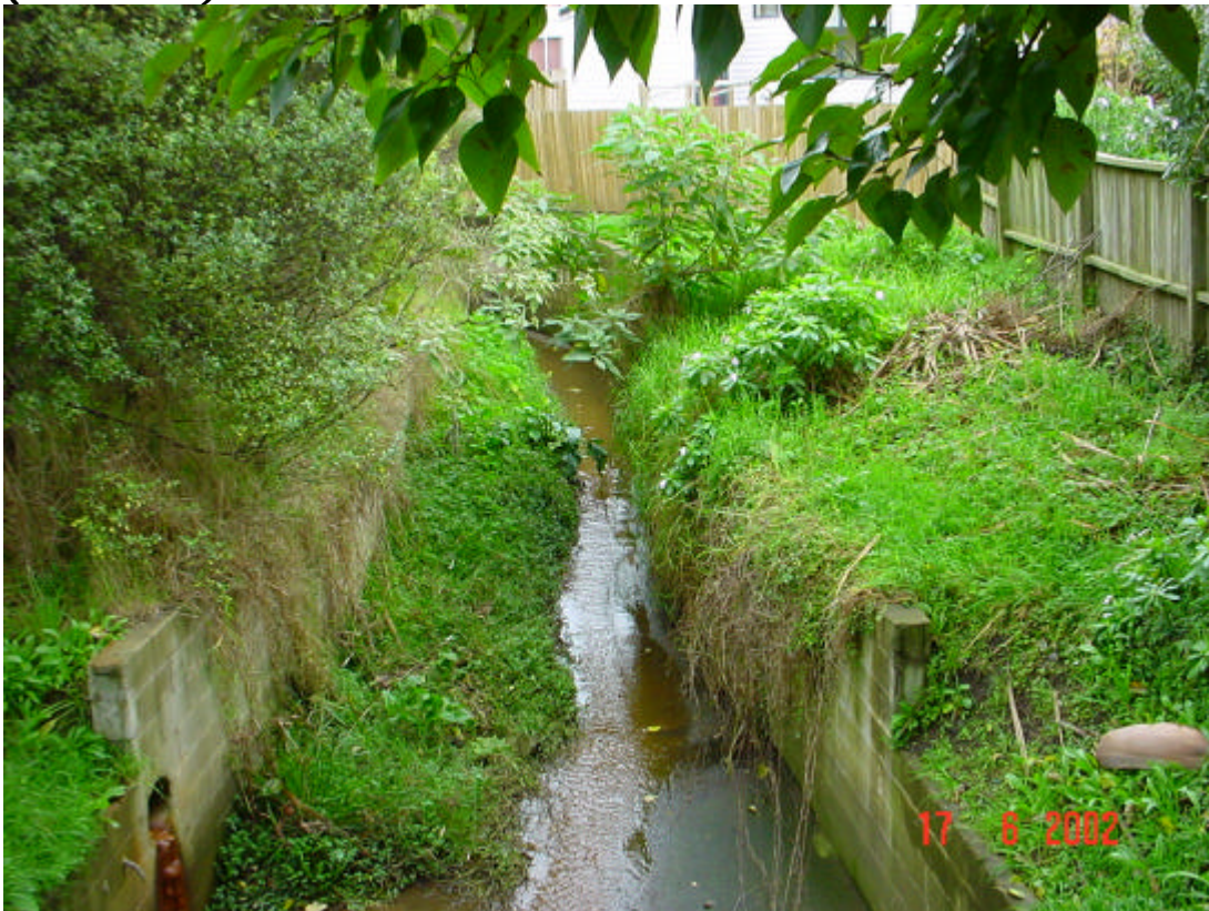
Figure J18: Stream Channel Between 90 and 104 Felton Matthew Avenue (June 2002)
