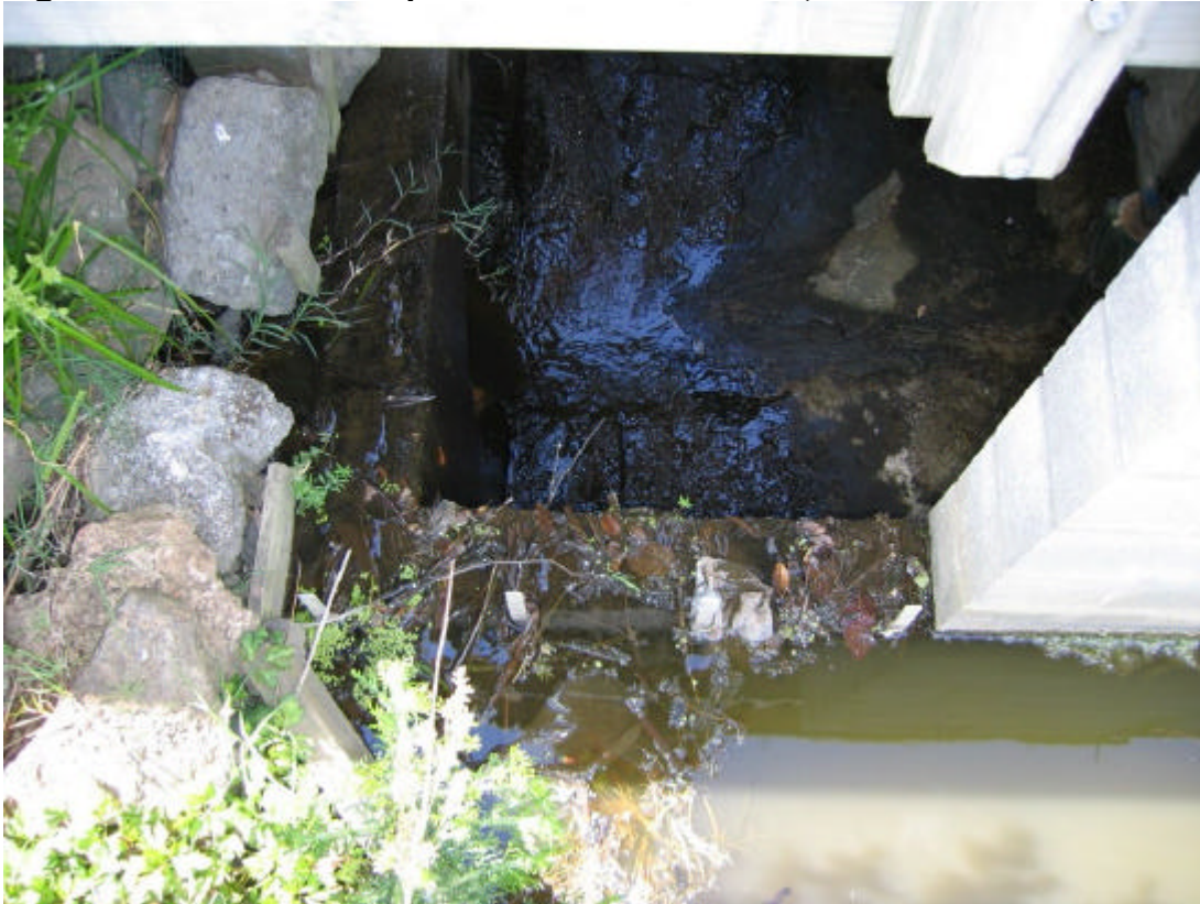
Figure J9: Tamaki Campus Pond Outlet Weir (December 2003)
