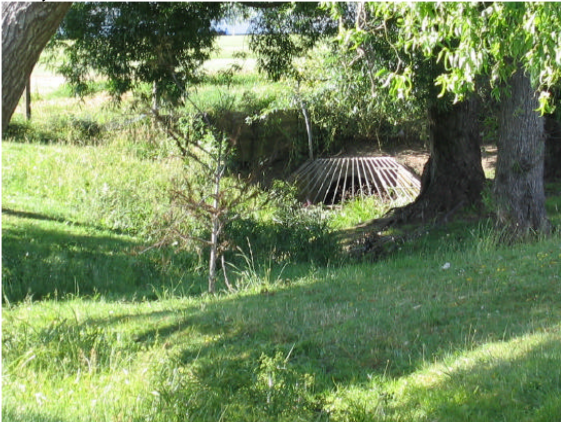
Figure J11: Inlet on Northern Boundary of Tamaki College (December 2003)
