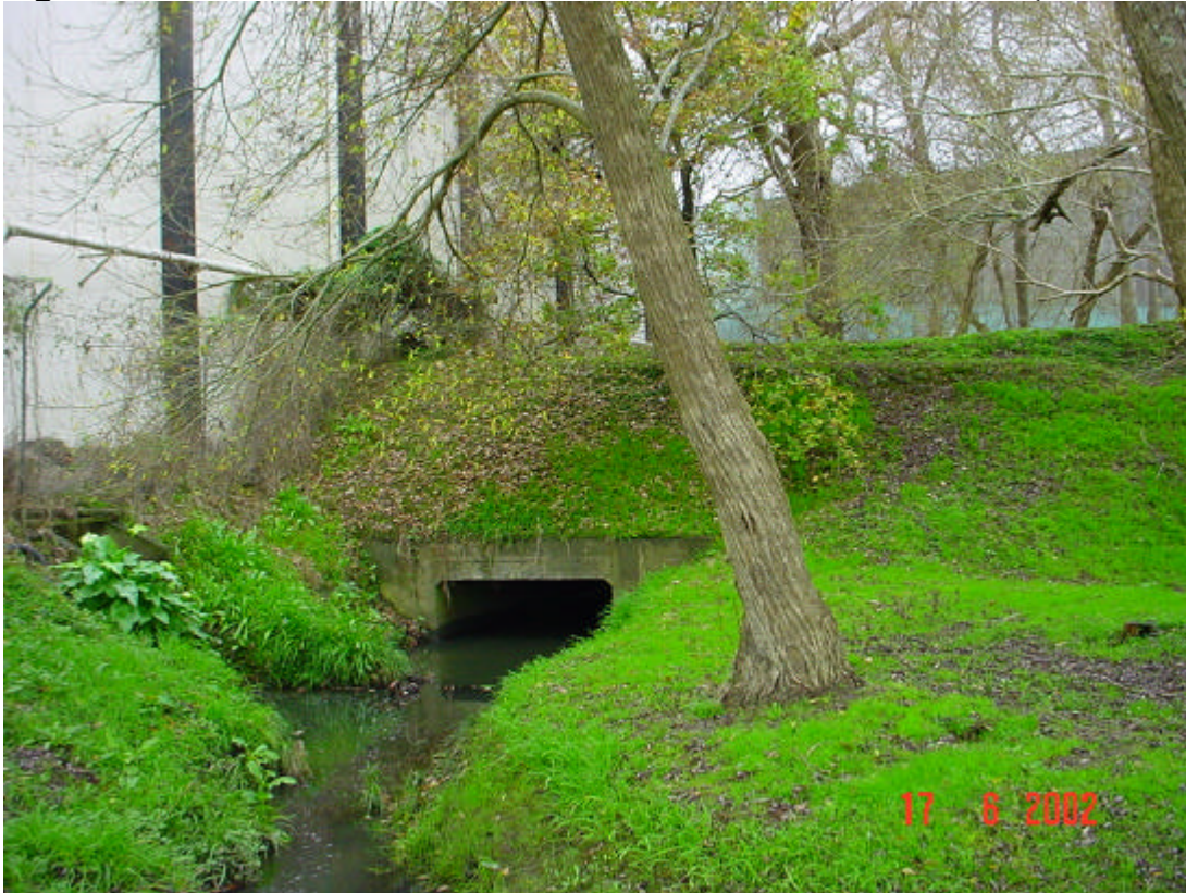
Figure J17: Eastview Reserve Bund and Culvert (June 2002)
