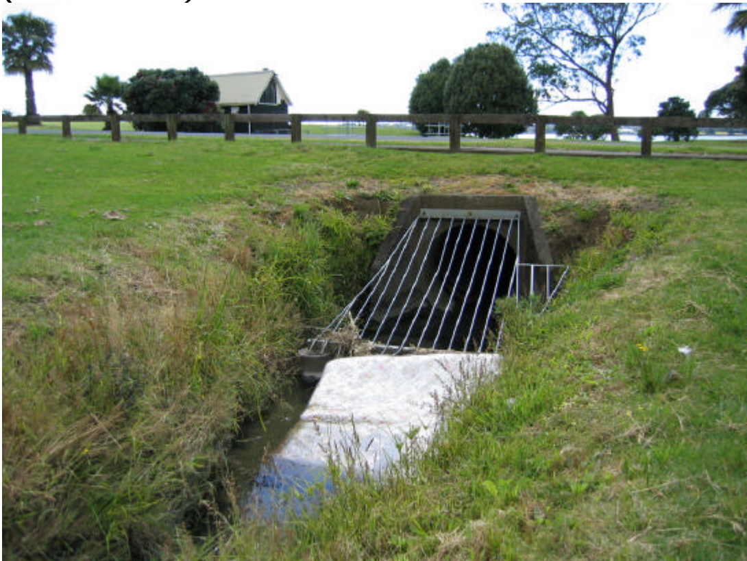
Figure J12: Culvert North of 115 Riverside Avenue (Boundary Reserve) (December 2003)
