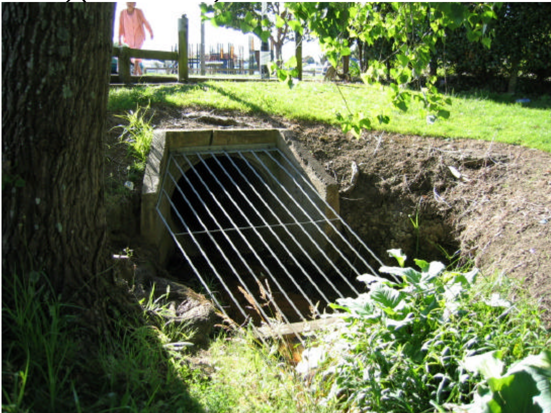
Figure J10: Culvert Between 45 and 47 Elstree Avenue (Wimbledon Reserve) (December 2003)
