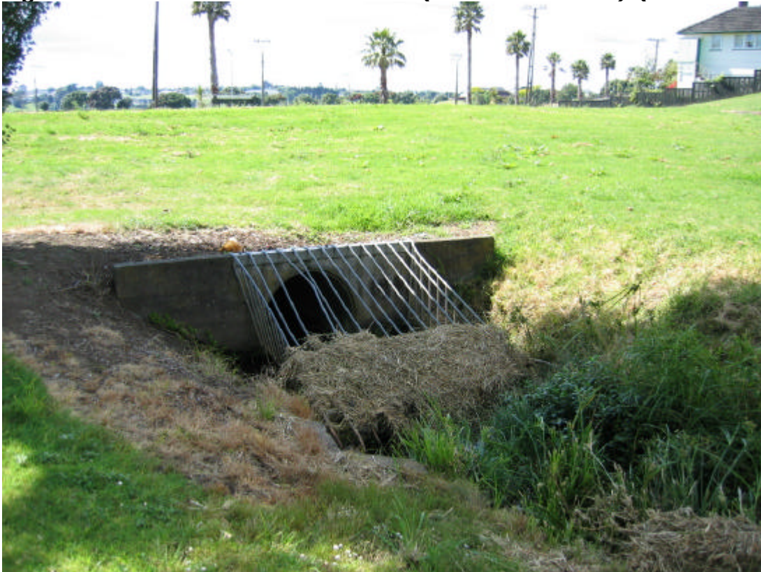
Figure J14: Inlet at 47 Dunkirk Road (Johnson Reserve) (December 2003)
