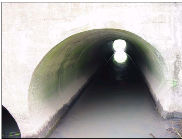
Figure 2.4 View from Downstream End before installation of gauge
