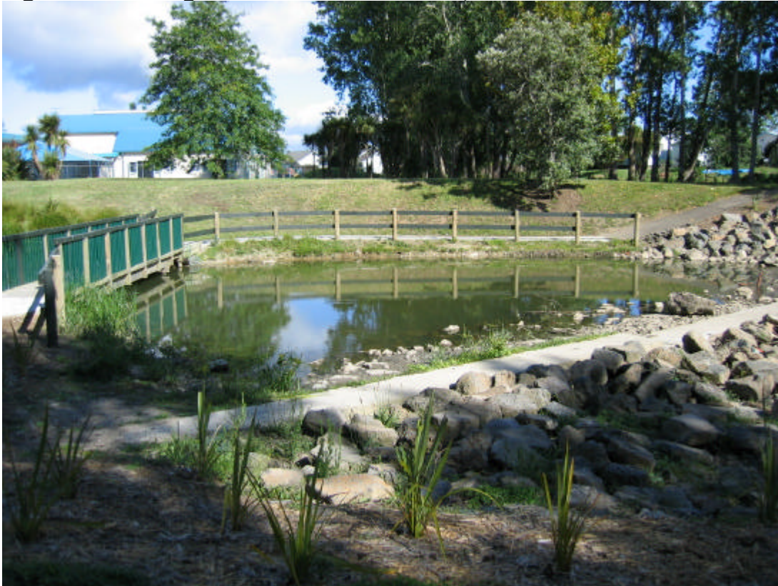
Figure J7: Pt England Pond Outlet Weir (December 2003)
