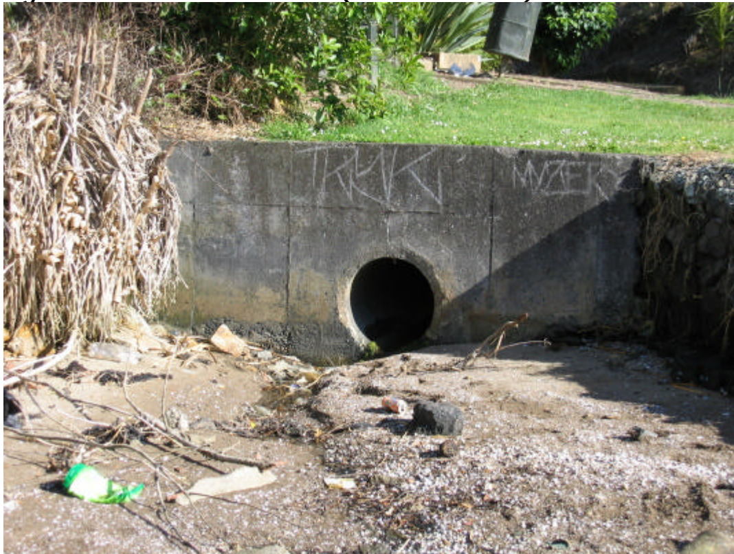
Figure J1- Tahaki Road Outlet (December 2003)
