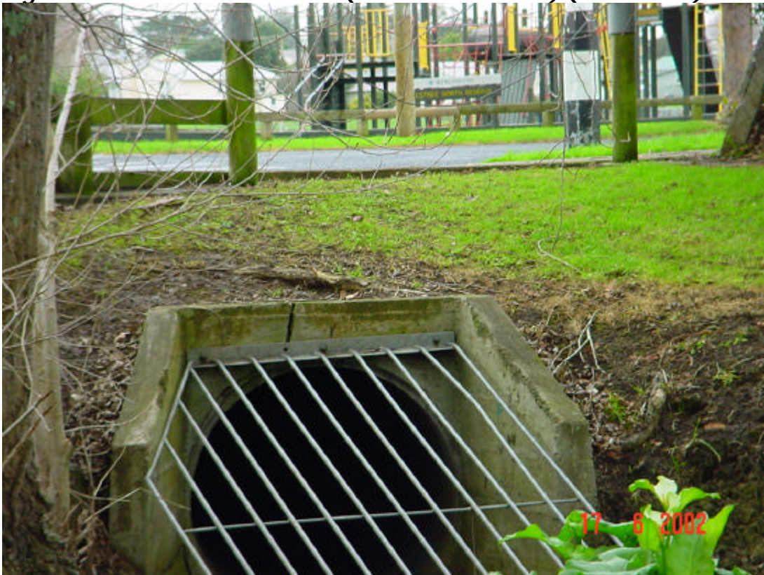
Figure J16: Line Road Culvert (Eastview Reserve) (June 2002)
