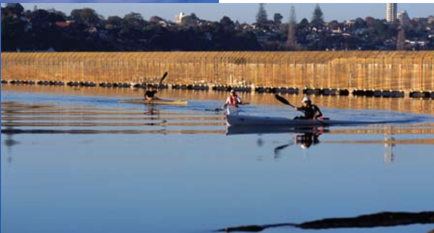
Watercare Project Hobson – removing the 90 year old sewer that bisects Hobson Bay and replacing it with a three kilometre tunnel will once again open up the bay for recreational use.
