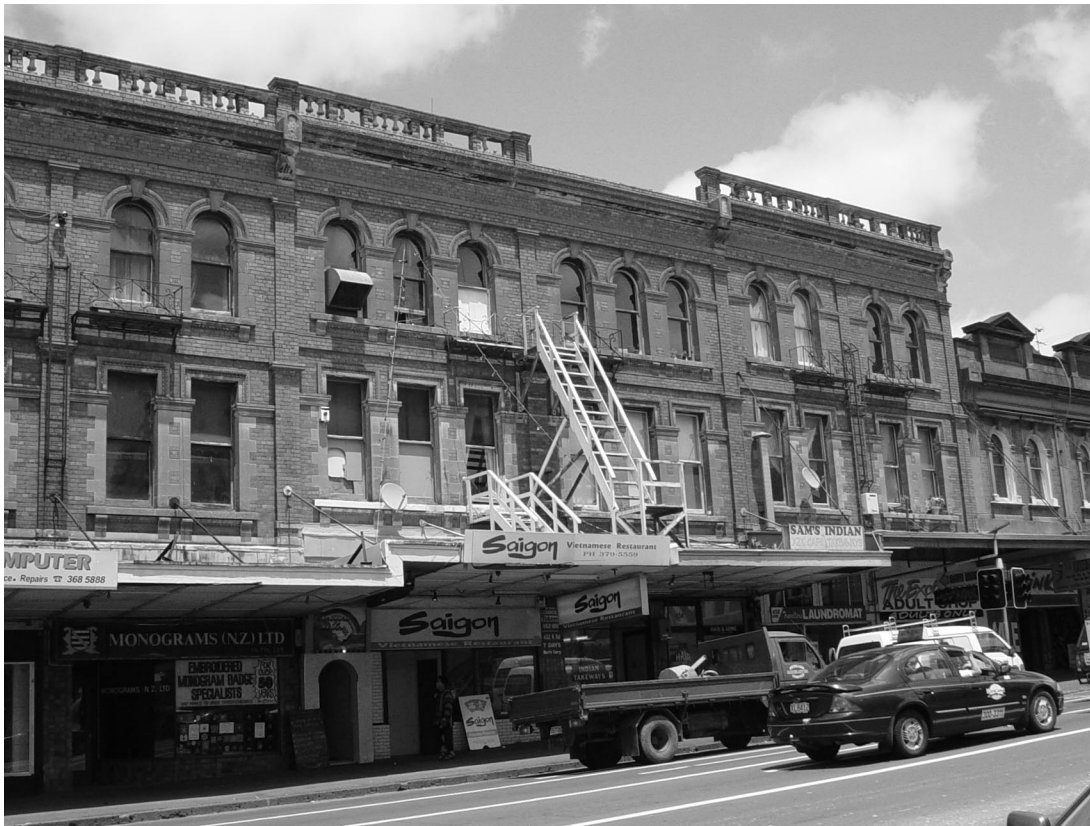
A “monolithic” frontage with narrow arched windows.
