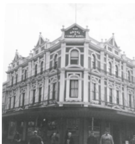
Division into bays, reflected particularly at the parapet
