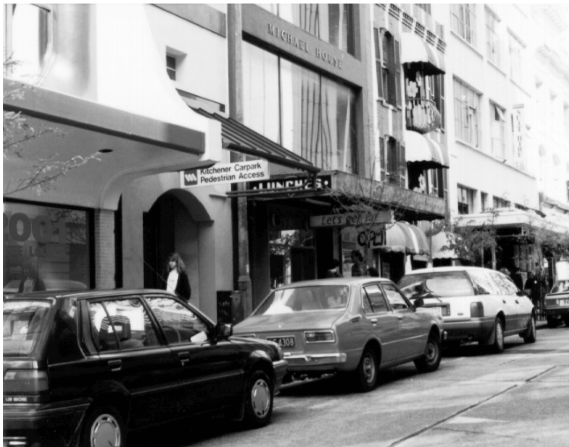
...High Street provides direct access to off-street parking in buildings fronting the street ...
