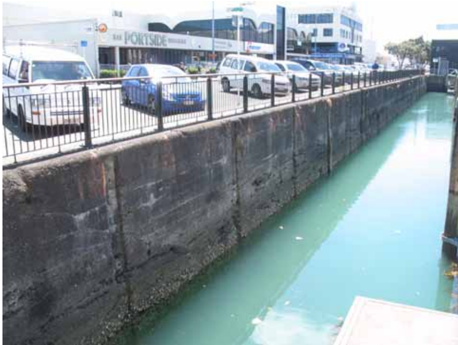
Intact section of Julian's wall, topped with modern balustrade. Note recesses for fender piles and ladders.
