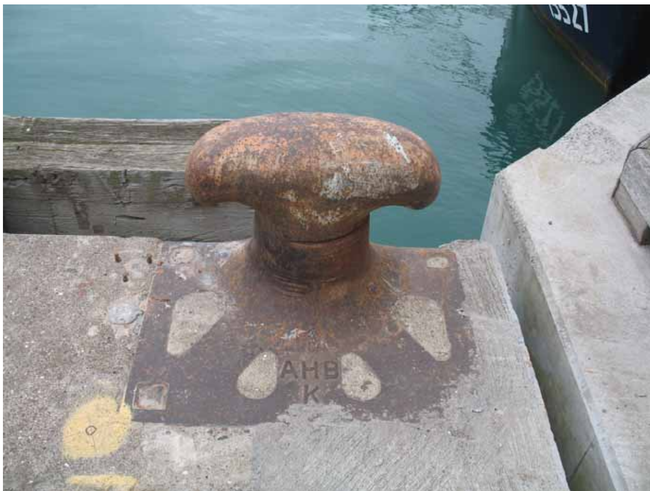
Type K bollard at eastern end of North wharf. Note textural difference between exposed aggregate surface of the historic wharf (far left) and modern wharf to right.
