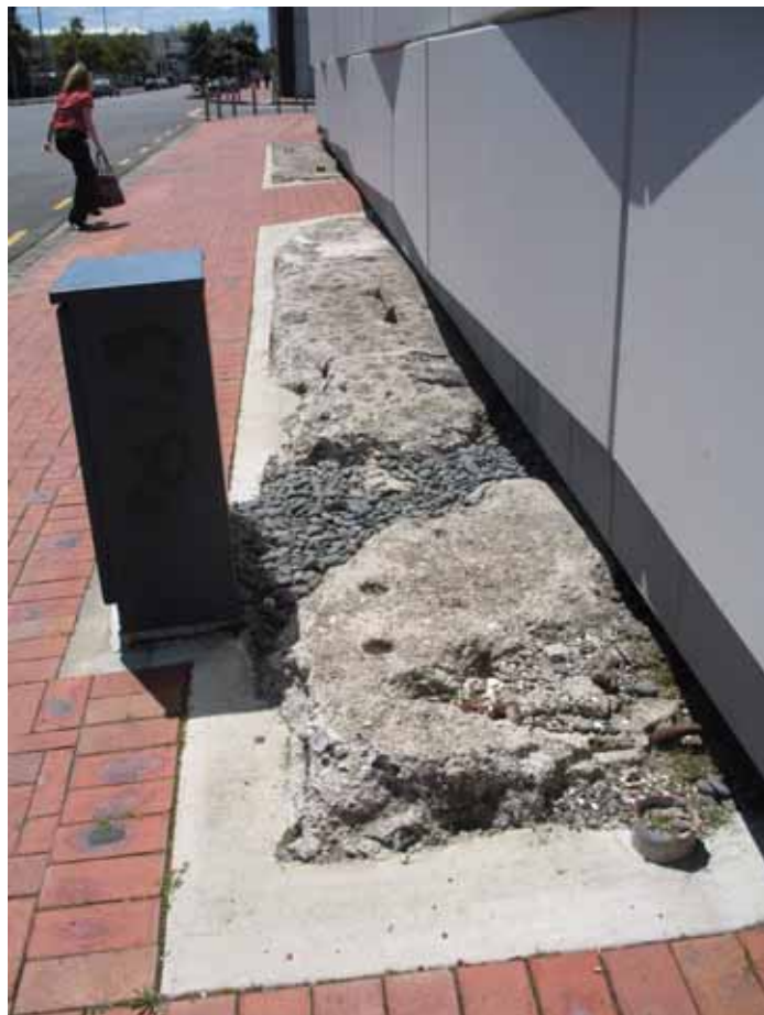
Sections of the top of Julian's wall that have been retained during construction of modern footpath between Viaduct Harbour Ave and Fanshawe Street.
