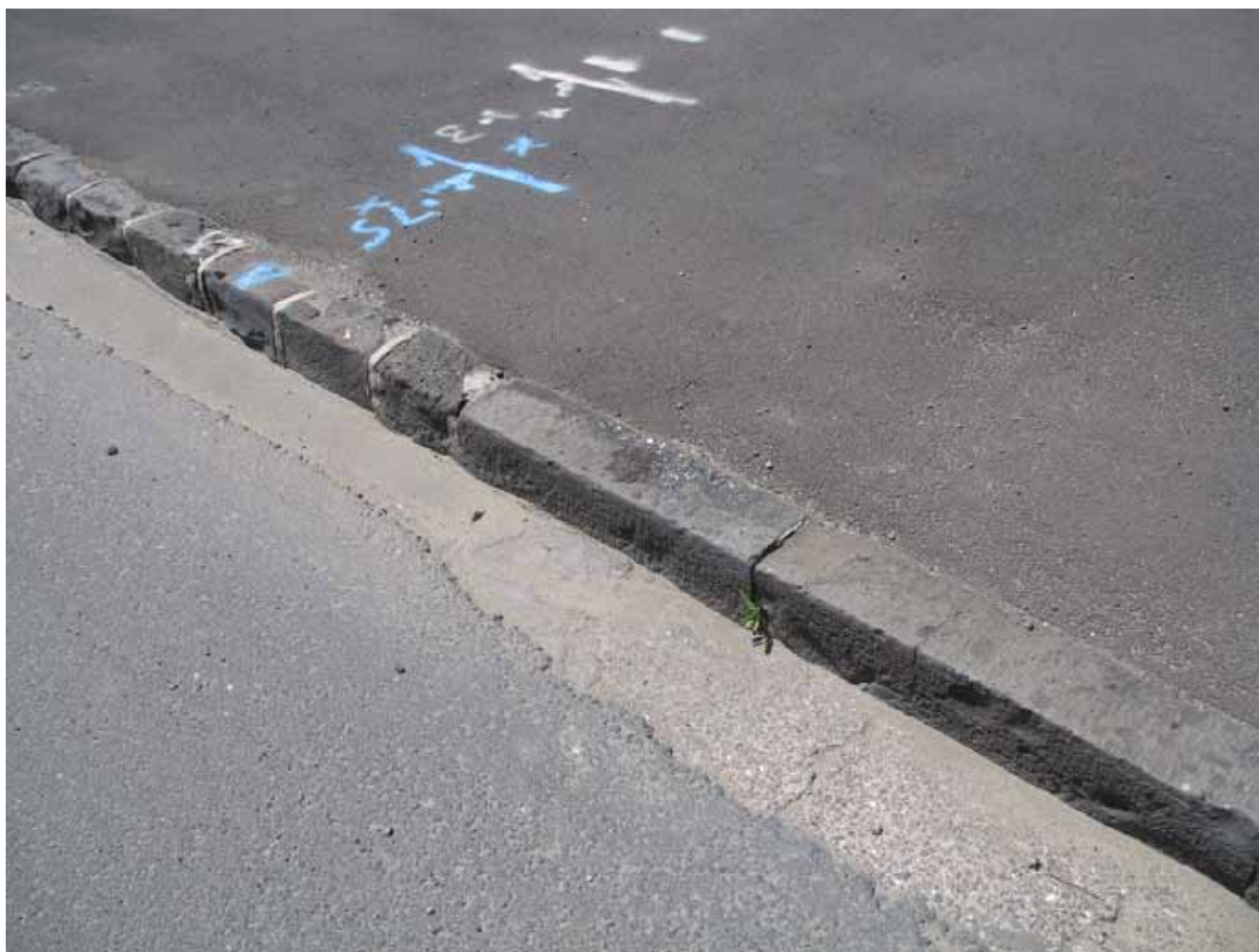
Bluestone kerbing , Beaumont St: Kerbing with original stones & detail on right, modern replacement on left.
