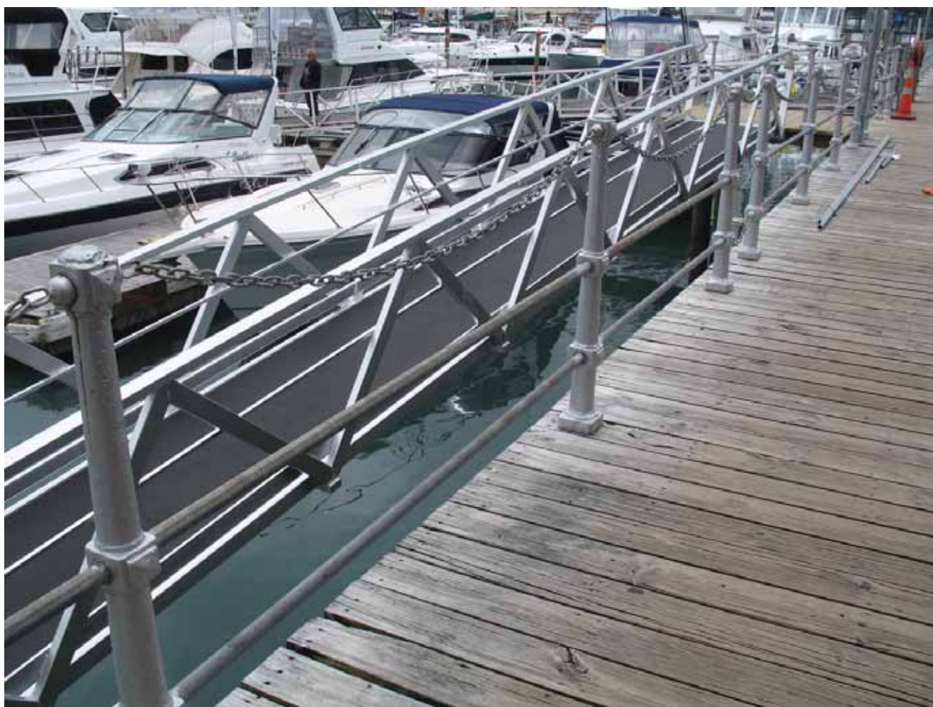
Modern balustrade incorporating recycled stations, Pier 21.
