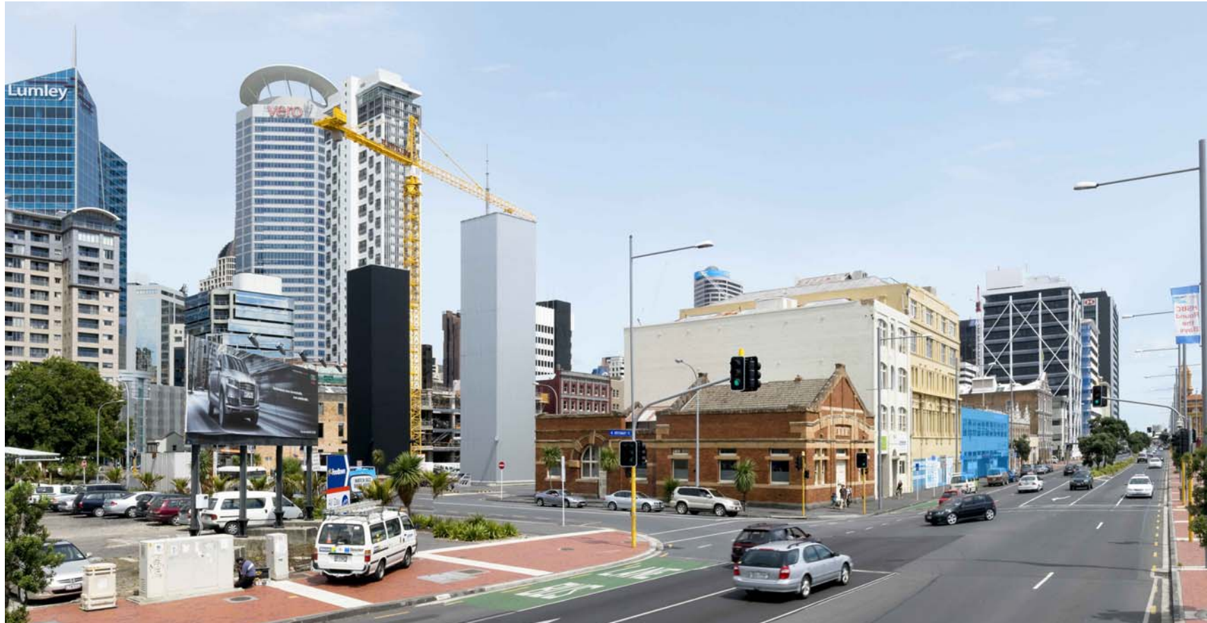
Figure 7: View towards Britomart looking west along Quay Street.
