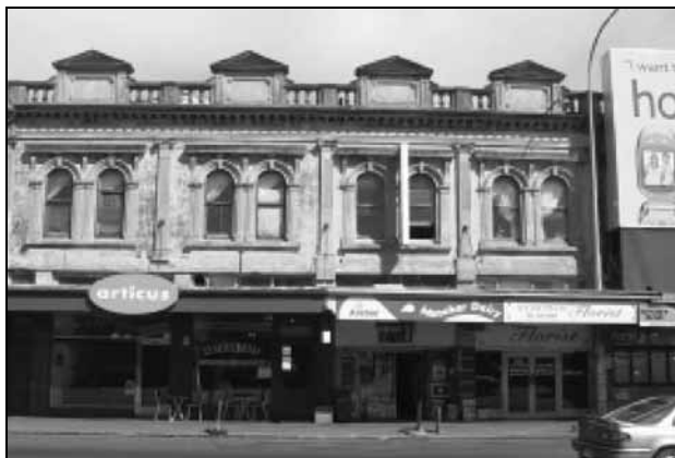
Solid plasterwork illustrating a variety of structural and ornamental motifs.
