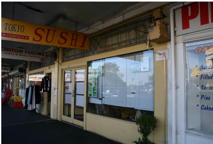
Original shop front detail remains including leadlight top lights, and timber window joinery.
