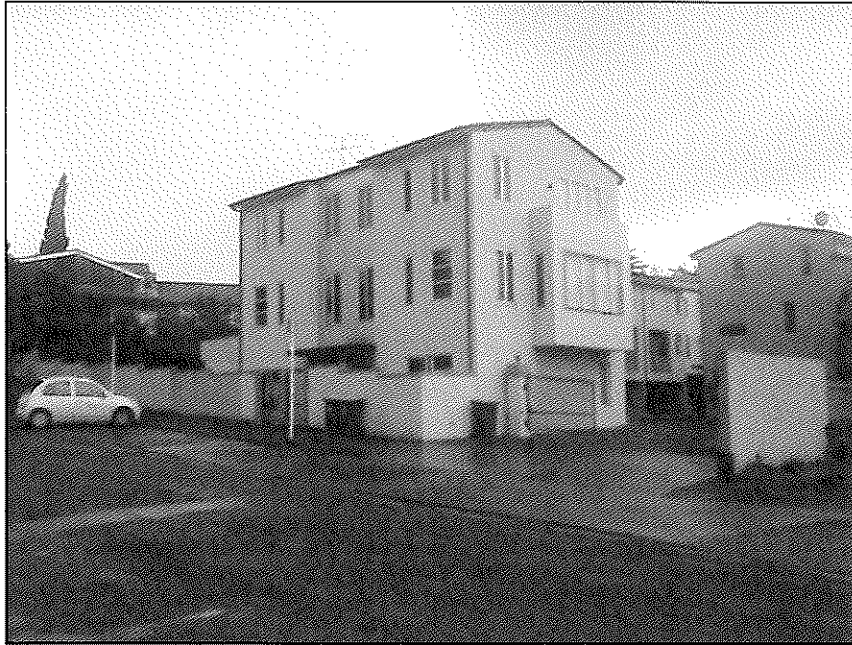
Figure 6: Example of High Density housing on Carlton Gore Road
