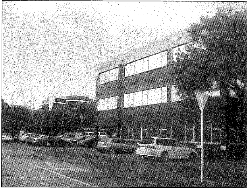
Figure 2: Photo of Subject Site (viewed from western boundary)
