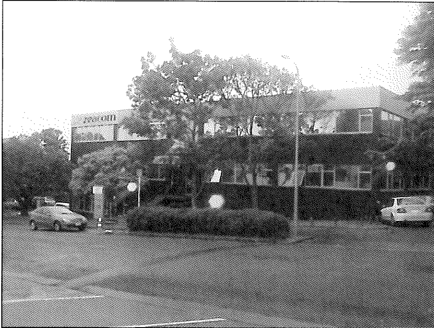
Figure 1: Photo of Subject Site
