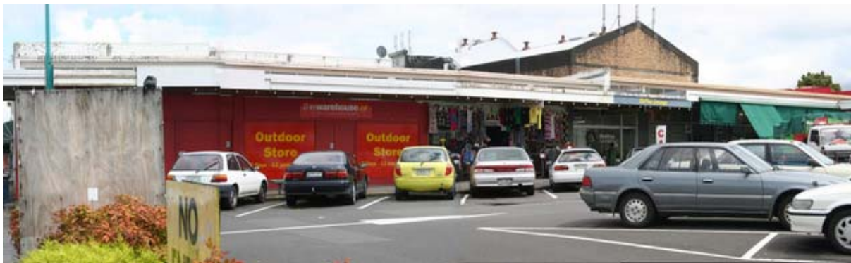
Photo 2: Rocklands Avenue entrance to TWL site
