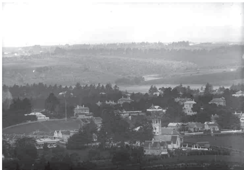
Figure 2. South west side of the church and the Priory from Mt Eden, showing the small outbuildings behind the house, ca. 1900. (Sir George Grey Special Collections, Auckland City Libraries, W140).
