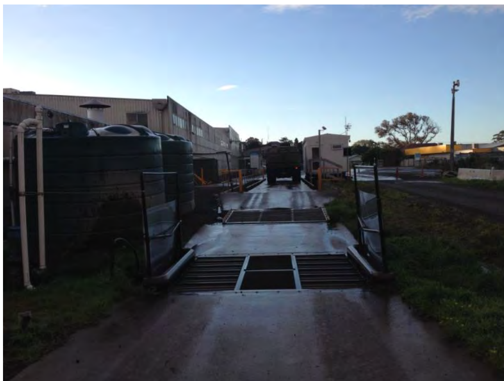
Photograph 40: Wheel wash area facing east showing water storage tanks for wheel wash water (left) and weighbridge / wheel wash (centre).
