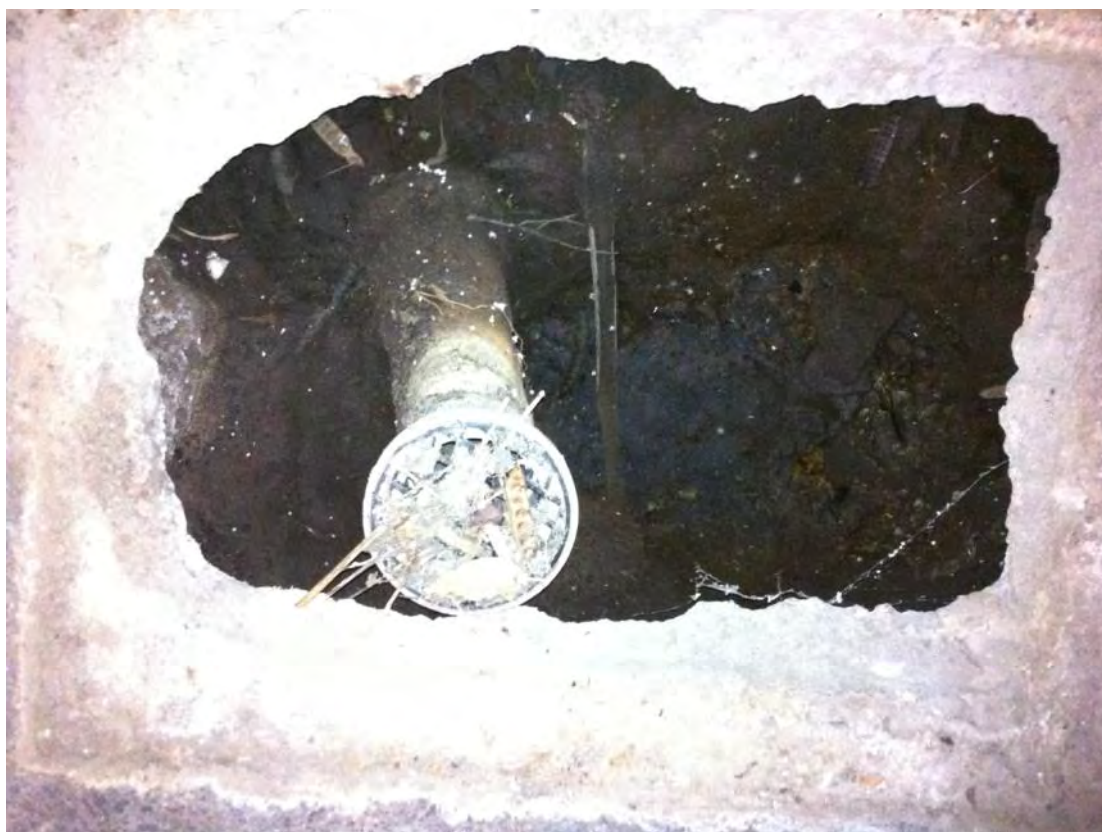
Photograph 18: Soakage pit inside the western building currently vacant.
