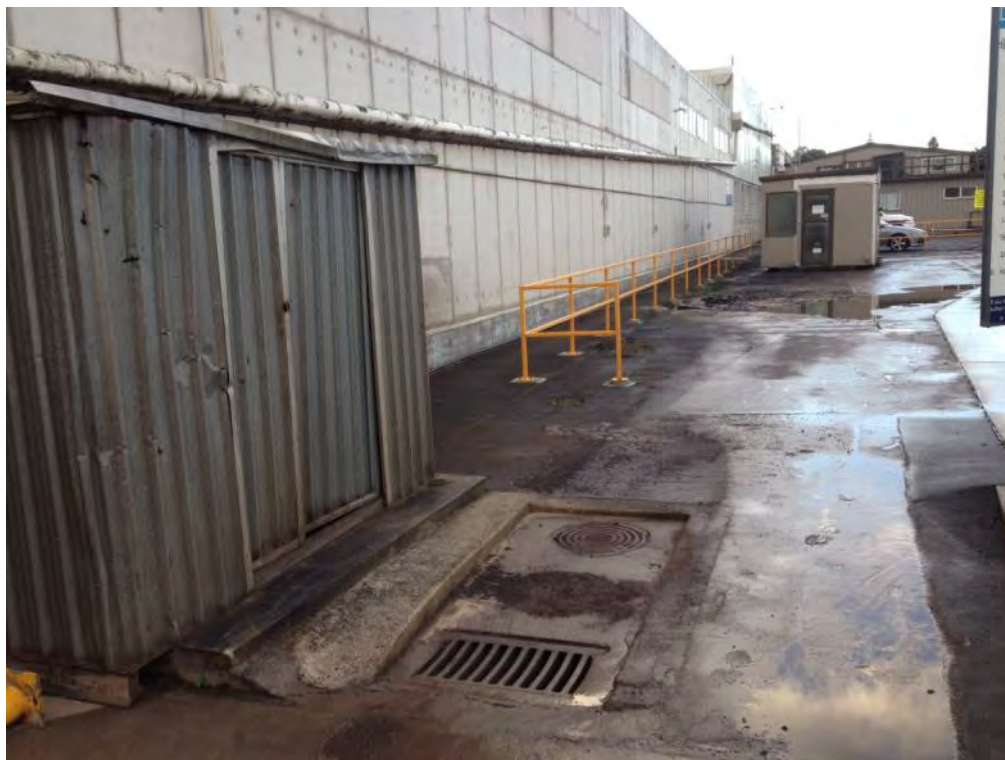
Photograph 41: Adjacent to the wheel wash and weighbridge area showing cesspit and interceptor; northern site boundary is indicated by the building on the left.
