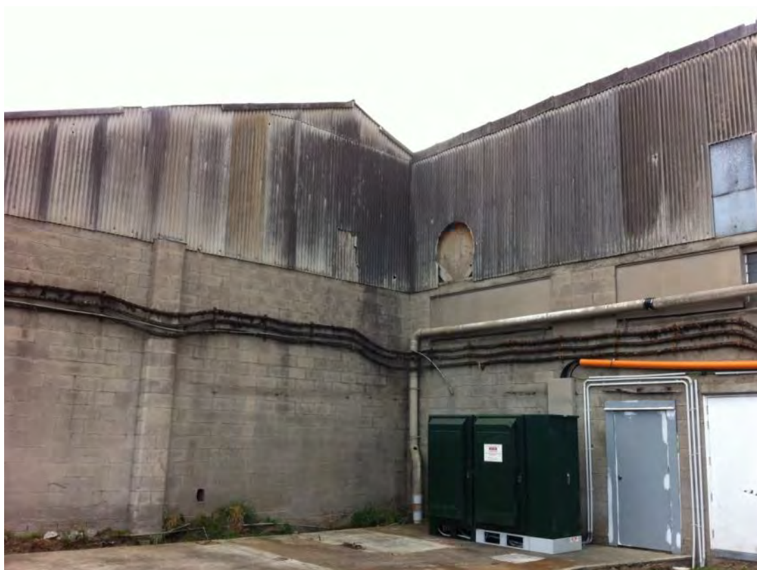
Photograph 22: Suspected ACM cladding on the southwest part of the main building complex.
