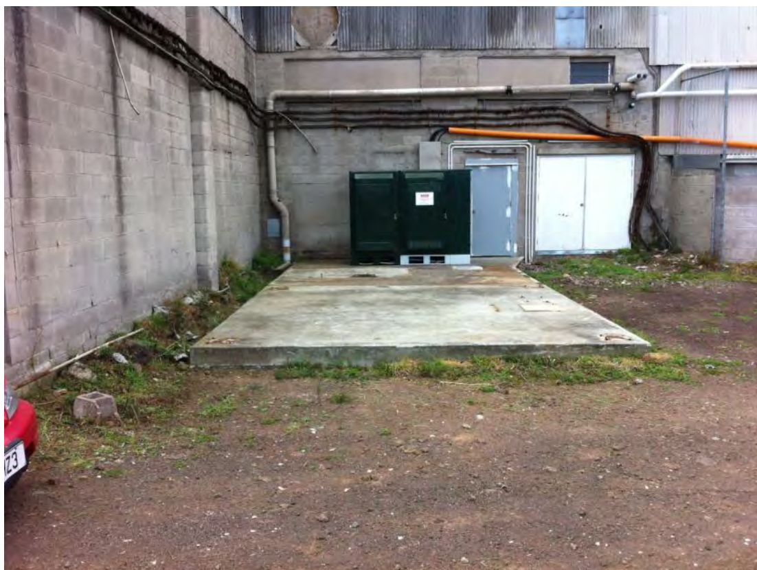
Photograph 20: Concrete pad for former dust extraction equipment.
