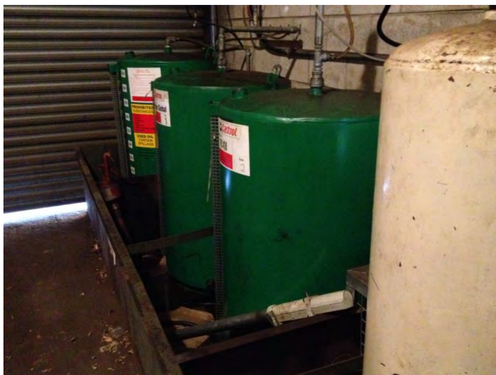
Photograph 34: Inside the engineering workshop showing banded oil storage area – both new and used hydraulic oils. Note: concrete floor.
