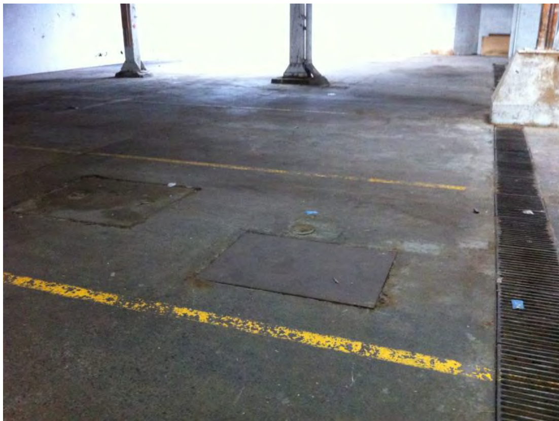
Photograph 17: Floor drains and metal covers over
