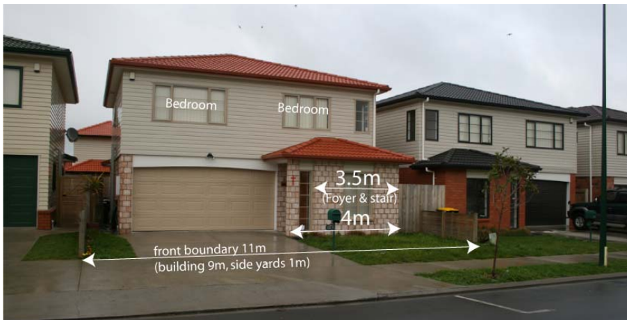
Example where no habitable ground floor rooms front the street, Mayfield Crescent, Flat Bush
