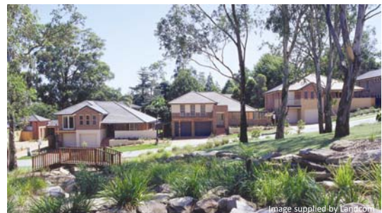
A good example where the change in level has been accommodated within the building
