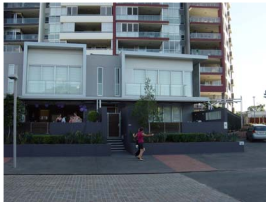
Street frontage with individual access to ground floor apartments in Brisbane.
