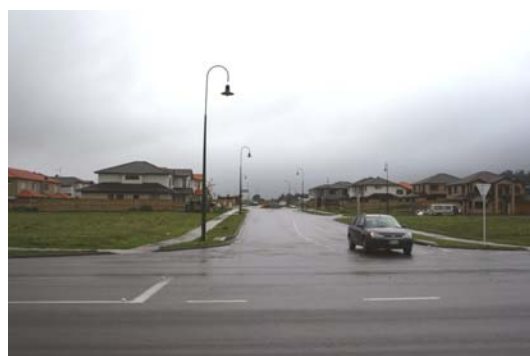
Erica Road (local road) existing with restrictions
