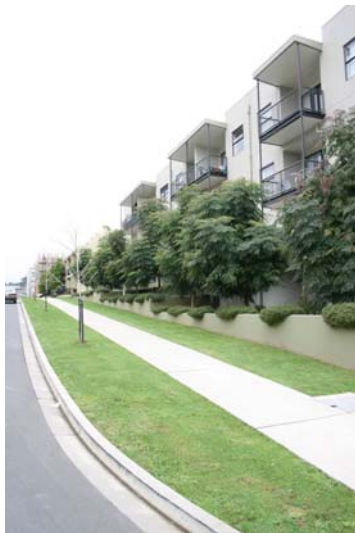
No access from the street frontage in Carlos Drive
