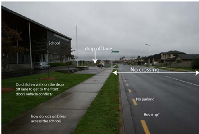
Existing situation at Baverstock School
