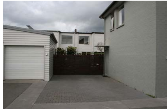
Rear lane detail at Addison, note wider permeable fence
