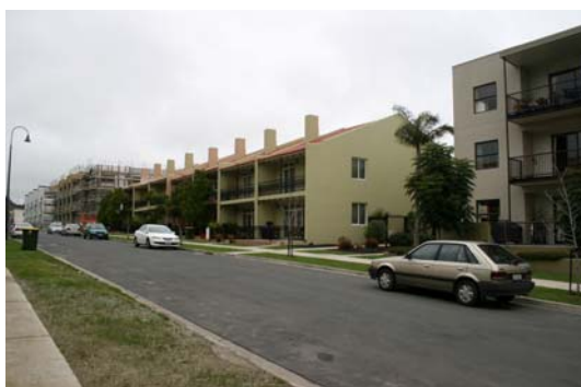
Mix of building typologies on Carlos Drive
