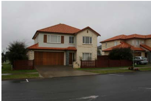
Single door double garage dominates the front yard
