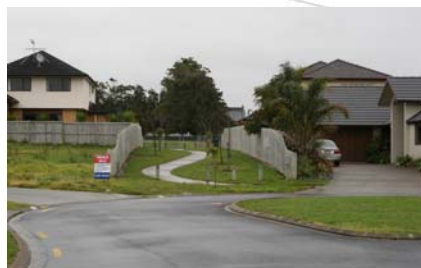
Existing pedestrian and cycle link with no frontage development
