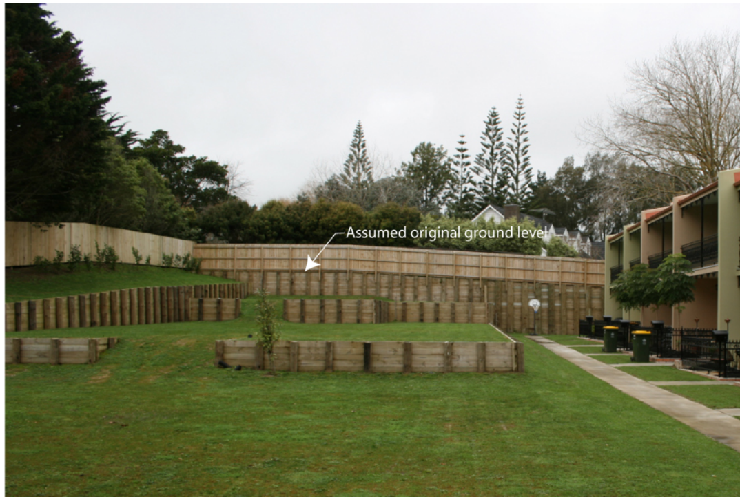
Illustration of excessive cut has been undertaken to provide a level building platform, Carlos Drive, Flat Bush
