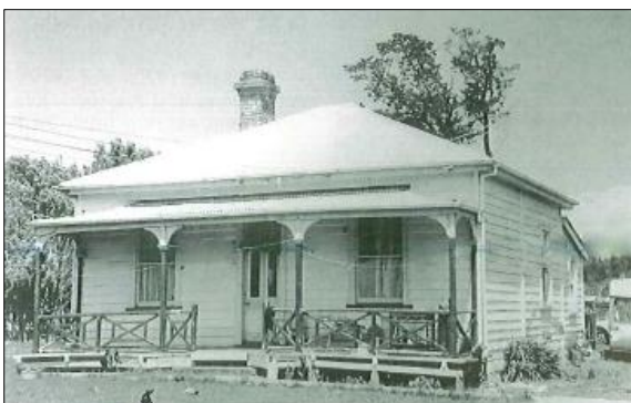
Fig 7: Murphy Homestead/ Flat Bush School house in 1997 when it still had its criss-cross verandah railing. Photo: Papatoetoe Historical Society
