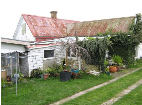
Fig 20: View from NE showing service lean-tos. Photo: Reynolds & Associates
