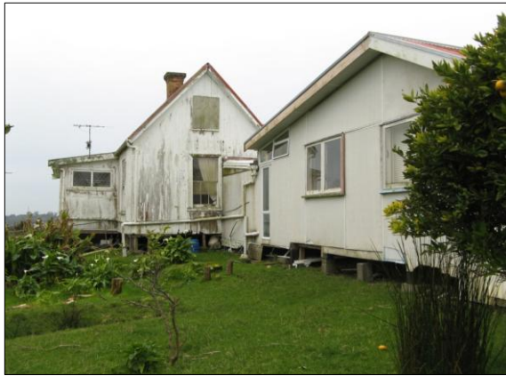
Fig 18 : South elevation showing addition. Photo: Reynolds & Associates
