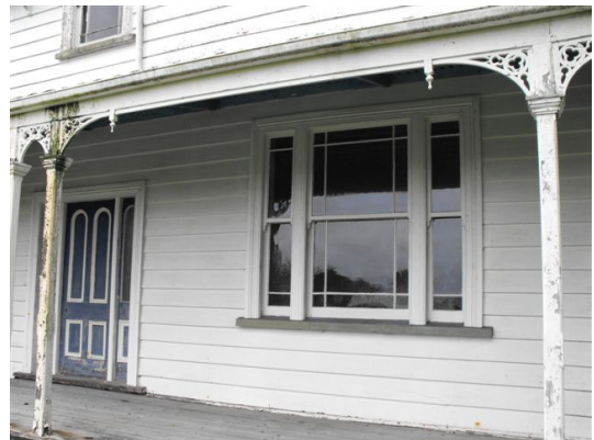
Figure 74: ‘Bordered’ Chicago window (ET Urban Design Ltd, 2010)
