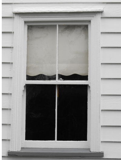
Figure 51: Four-paned window (ET Urban Design Ltd, 2010)
