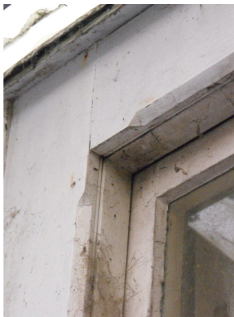
Figure 30: Chamfered detail (ET Urban Design Ltd, 2010)
