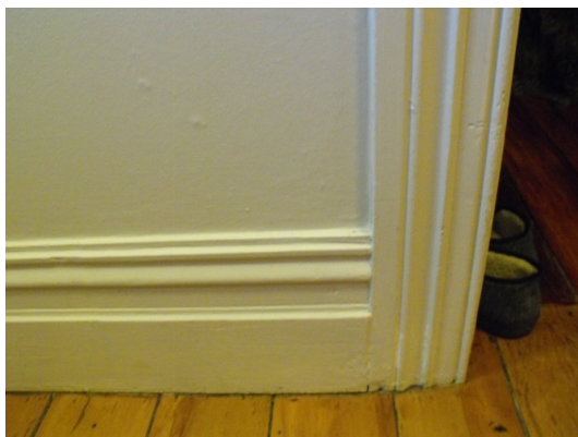
Figure 61: Timber skirting and architrave (ET Urban Design Ltd, 2010)
