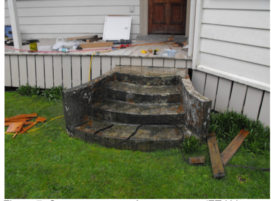
Figure 7: Concrete steps to front entrance (ET Urban Design Ltd, 2010)
