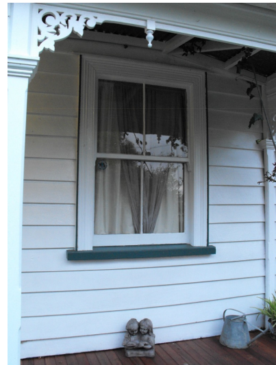
Figure 60: Front window and verandah detailing (ET Urban design Ltd, 2010)
