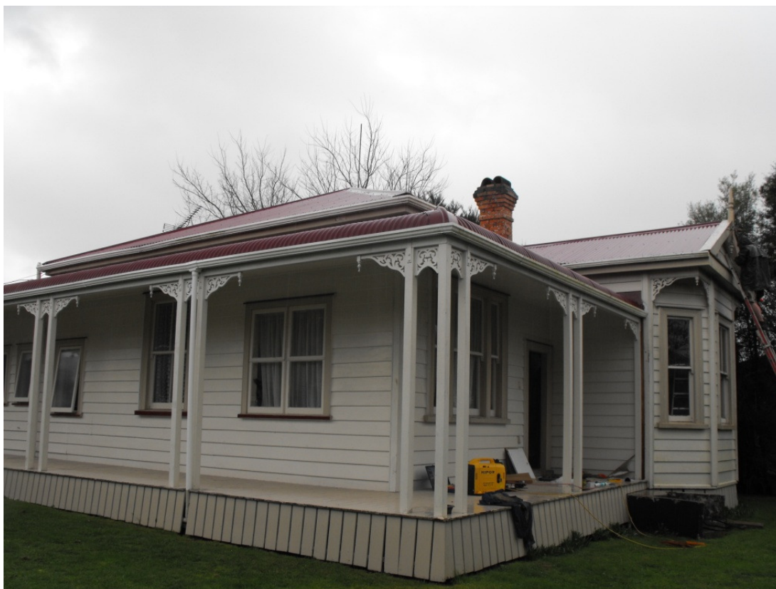
Figure 2: 1 Monument Road (ET Urban Design Ltd, 2010)
