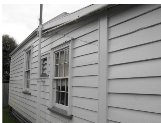
Figure 48: South elevation with line of original lean-to roof visible (ET Urban Design Ltd, 2010)
