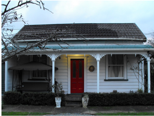
Figure 55: East elevation of main cottage (ET Urban Design Ltd, 2010)
