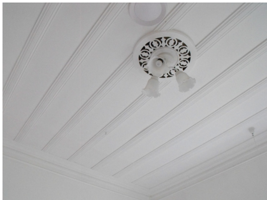
Figure 42: Board and batten ceiling with fretwork timber rose (ET Urban Design Ltd, 2010)
