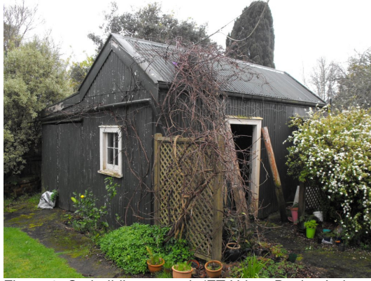
Figure 6: Outbuilding to north (ET Urban Design Ltd, 2010)
