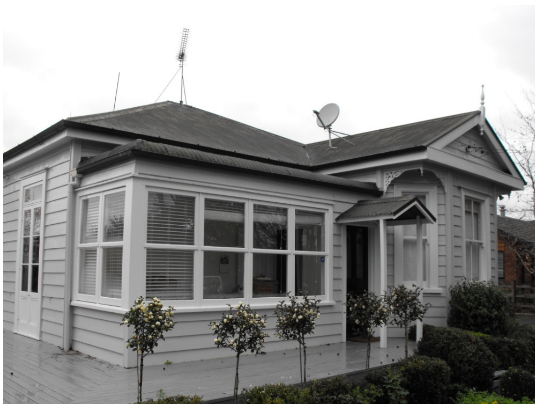
Figure 10: 8 Monument Road (ET Urban Design Ltd, 2010)
