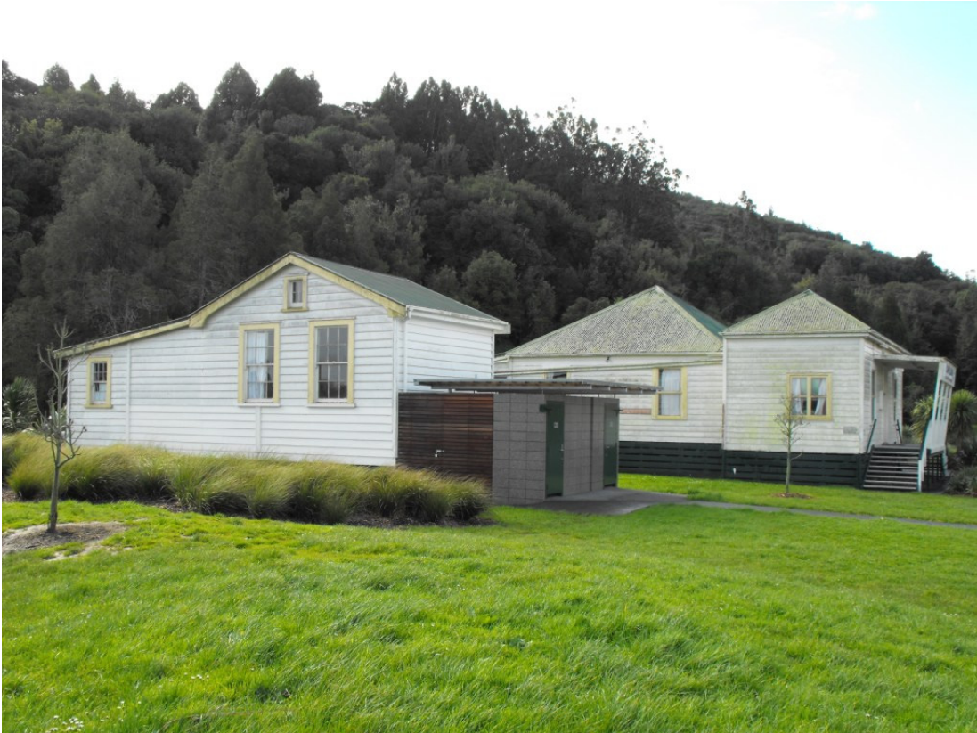
Figure 63: Camp Sladdin Complex, Thorps Quarry Road with former North School Building to left (ET Urban Design Ltd, 2010)
