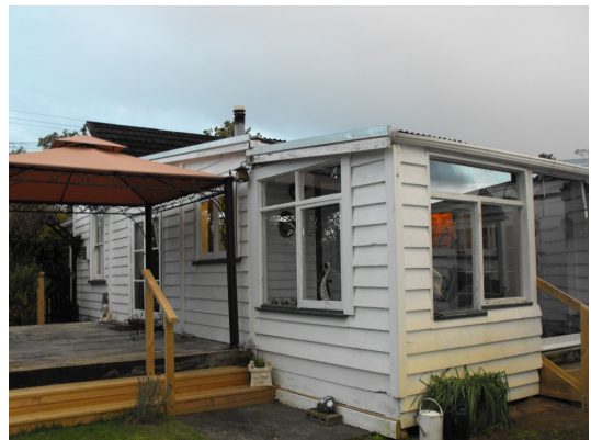
Figure 58: View from north-west (ET Urban Design Ltd, 2010)
