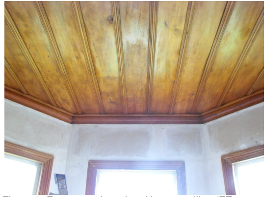
Figure 9: Front room board and batten ceiling (ET Urban Design Ltd, 2010)
