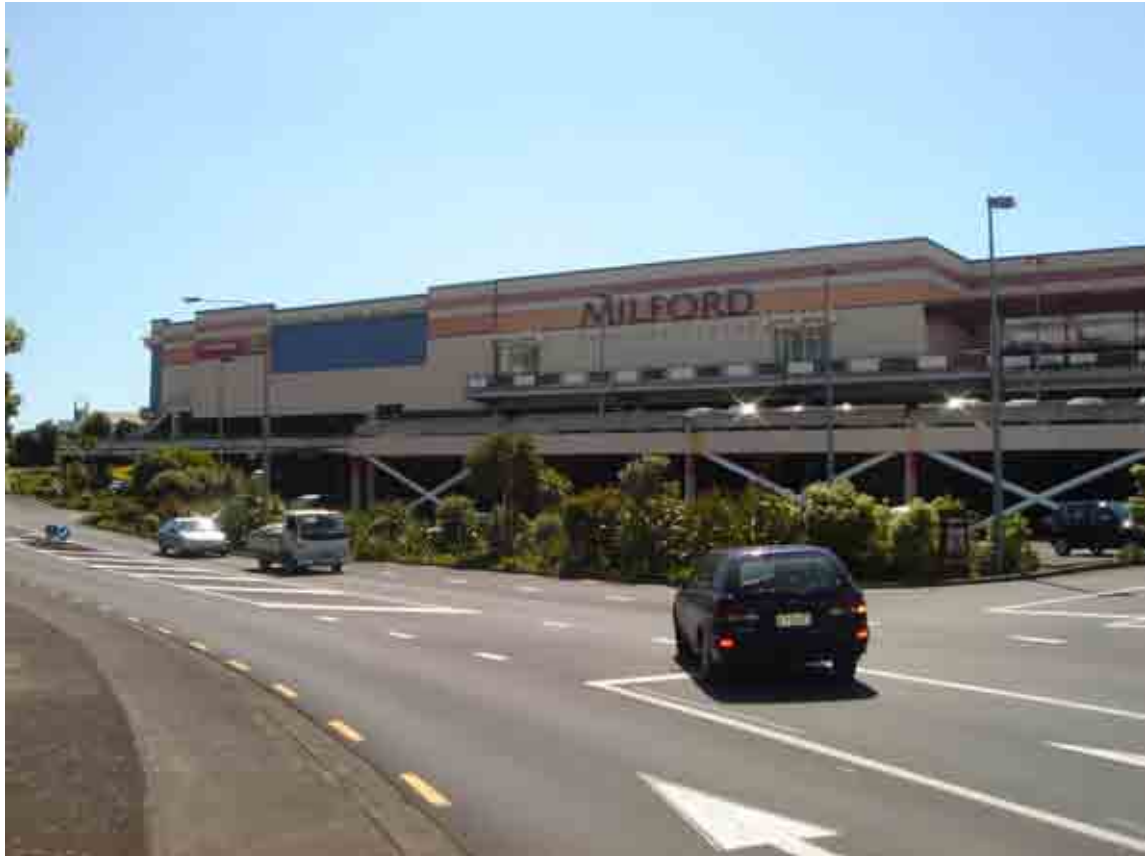
Photograph 5: The western façade of the Milford Shopping Centre
