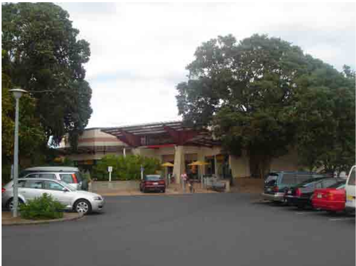
Photograph 2: Milford Shopping Centre buildings to the south of the car park
