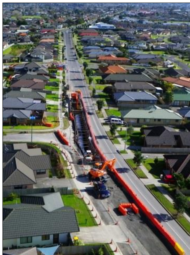
Figure 6: example of construction area with traffic management
