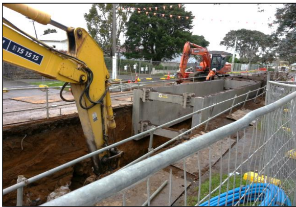
Figure 4: trench being dug in road
