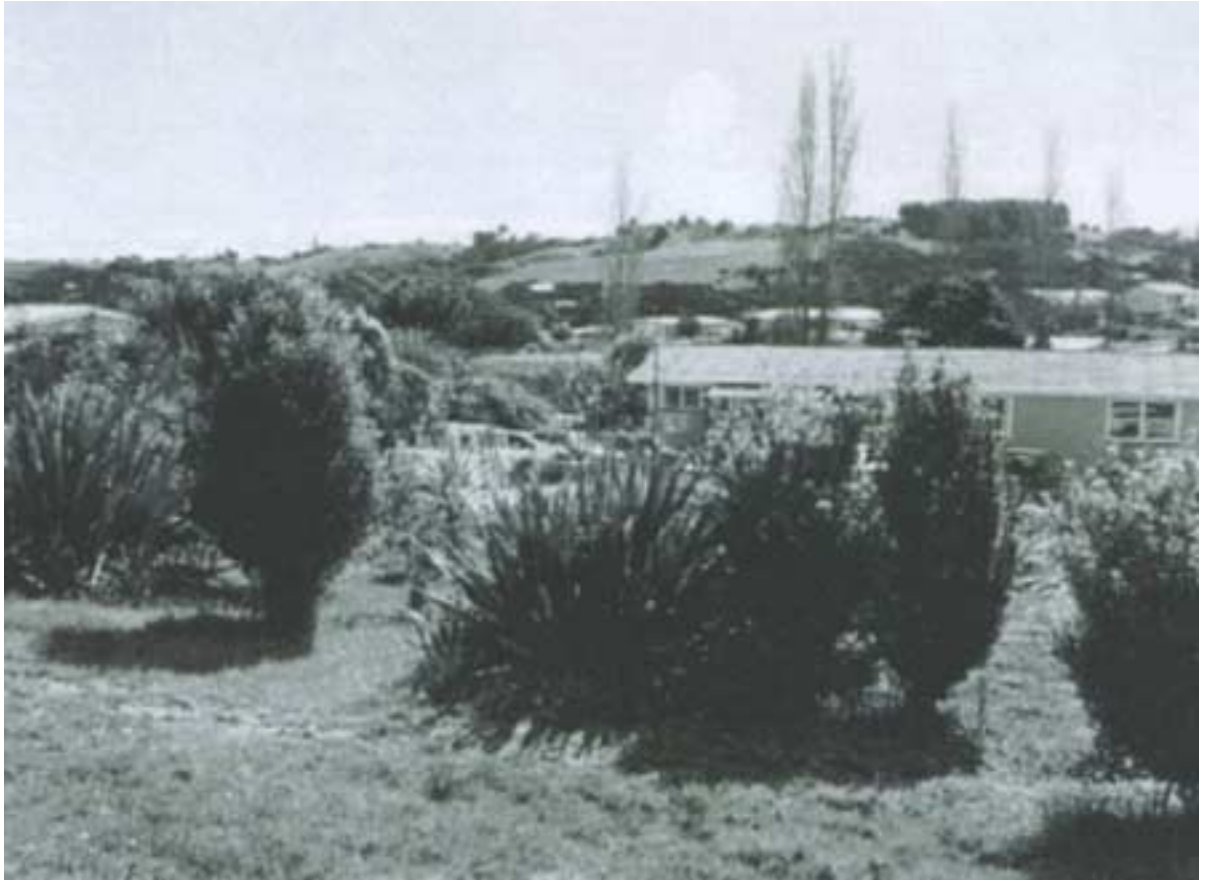
Figure 6 The Catherine Mitchell hall is visually well integrated
