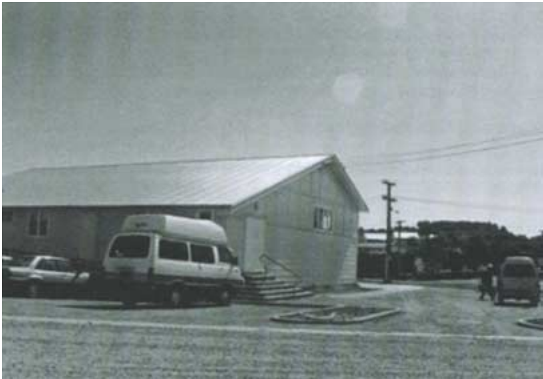
Figure 10 Existing provision for car parking is adequate most of the time
