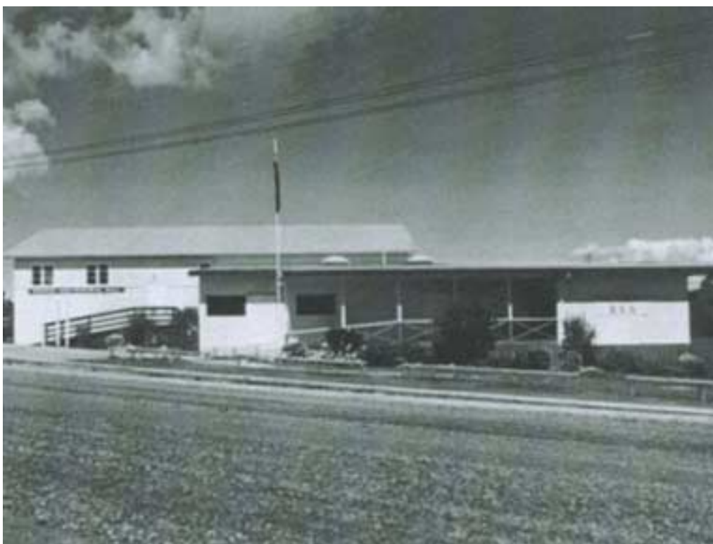
Figure 1 Anzac Reserve houses the Waiheke War Memorial Hall and RSA
