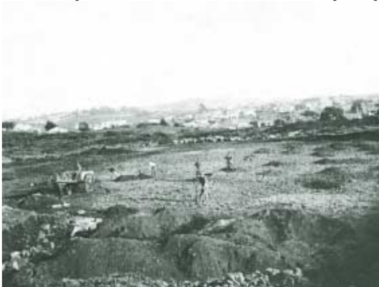
Figure 2 Bowling Greens being formed
