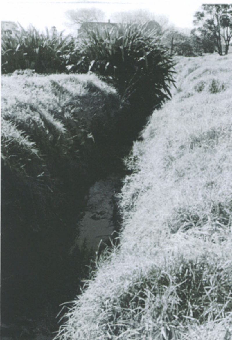
Figure 8 The storm water drain to be rehabilitated
