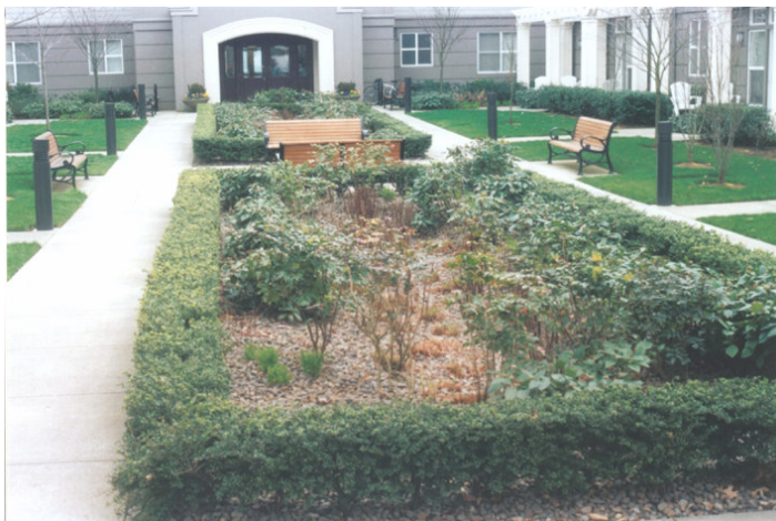
Photo 5 Stormwater Planter: Sunken Type
