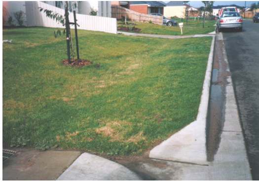
Photo 6 Grass Swale on Urban Street
