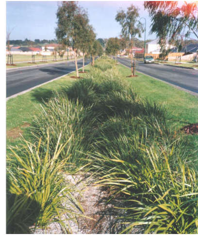
Photo 7 Swale & Gravel Trench System on Divided Road
