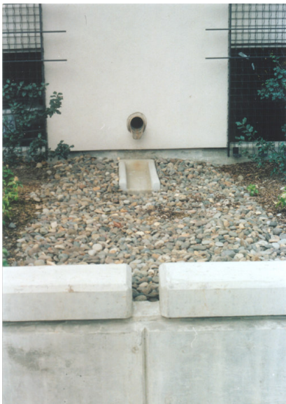
Photo 4 Stormwater Planter: Above- Ground "Rock Garden" Type
