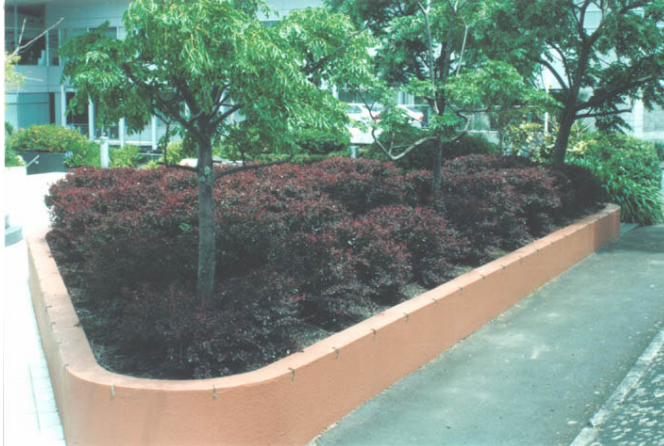
Photo 3 Stormwater Planter: Conventional Above-Ground Type
