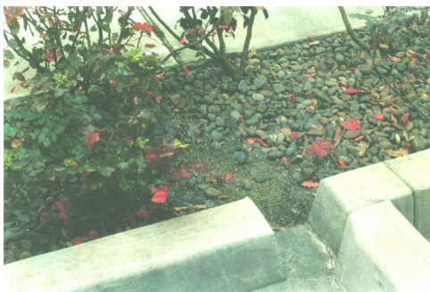
Photo 10 Car Park Kerb-Cut (feeding gravel swale)
