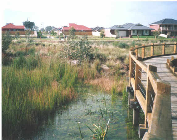
Photo 13 Wet-Type Detention Pond
