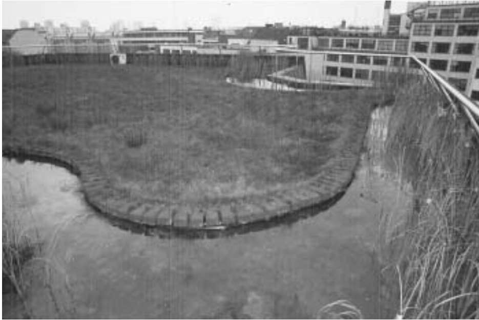
Plate 12-4: Wetland on a roof
