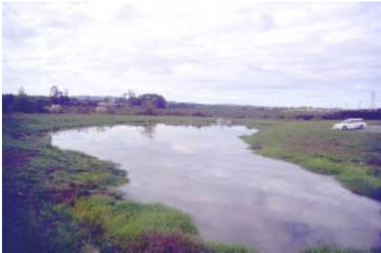
Plate 14-4: Example of a pond having a good shape but no provision for landscape planting
