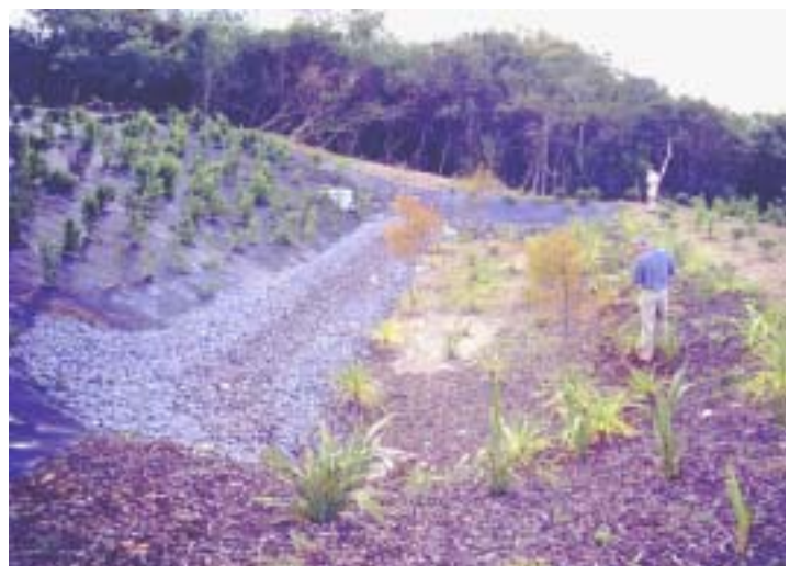
Plate 14-5: Example of a dry extended detention pond with good landscaping
