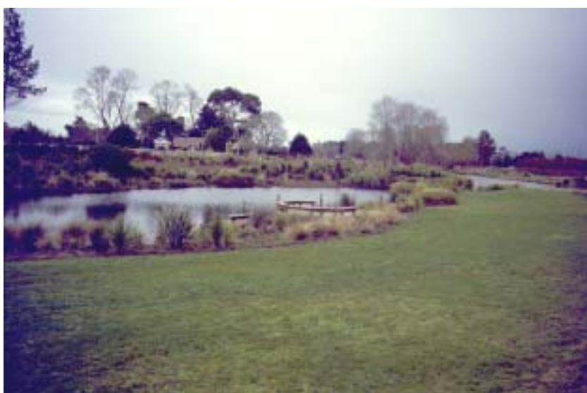
Plate 14-3: A well landscaped stormwater management pond
