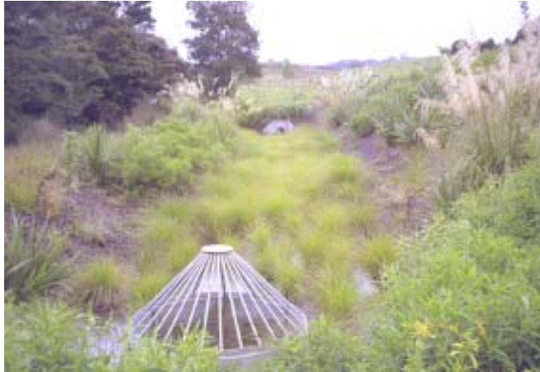
Plate 14-2: Stormwater management pond with significant landscaping
