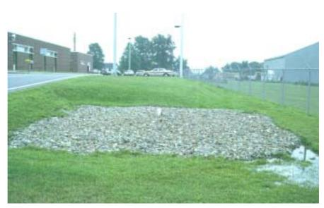
Plate 8-2: Infiltration trench with a swale for pretreatment
