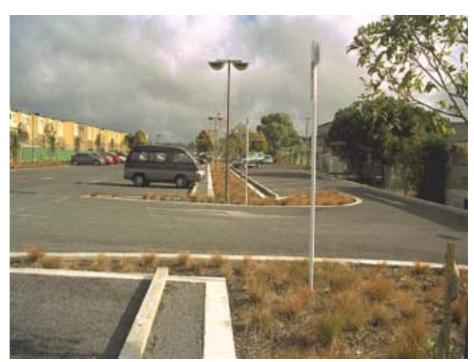
Plate 7-2: Example of a rain garden used in a parking lot
