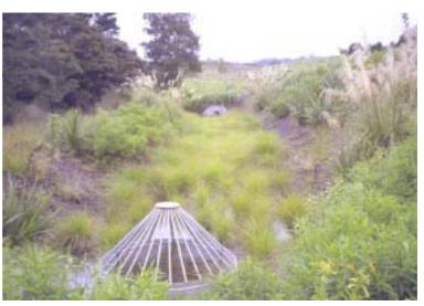
Plate 14-2: Stormwater management pond with significant landscaping
