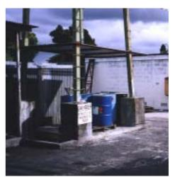
Plate 3-1: Chemical roof and bunding
