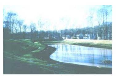
Plate 5-2: Example of a safety bench (above water) in conjunction with a shallow bench (note: normal pool level has been lowered to allow for planting of shallow bench)
