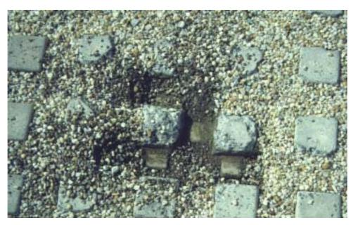
Plate 8-7: Modular paving with pea gravel filler
