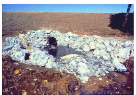
Plate 13-1: Example of riprap at a stormwater outfall
