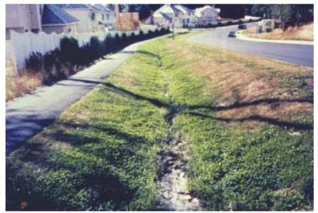
Plate 9-6: Swale needing maintenance due to high sediment loads
