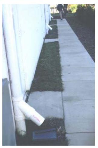
Plate 8-4: Infiltration dry well
