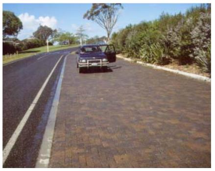
Plate 8-6: Example of a porous block parking area
