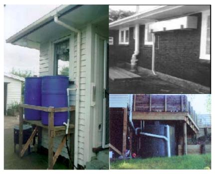
as multipurpose devices to provide treatment, peak attenuation and non-potable water supply benefits. They become financially self-supporting for reasonably large non-potable water demands when coupled with adequate roof areas
