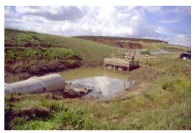
Plate 14-1: Example of a stormwater pond with little attention given to landscaping
