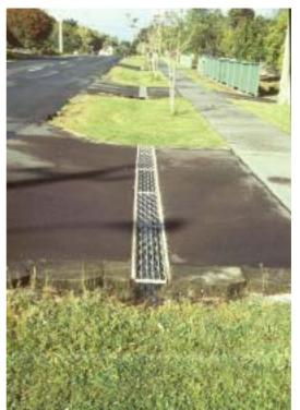
Plate 9-1: Example of a well designed and maintained swale
