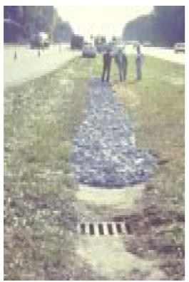
Plate 8-1: Infiltration trench treating roadway runoff
