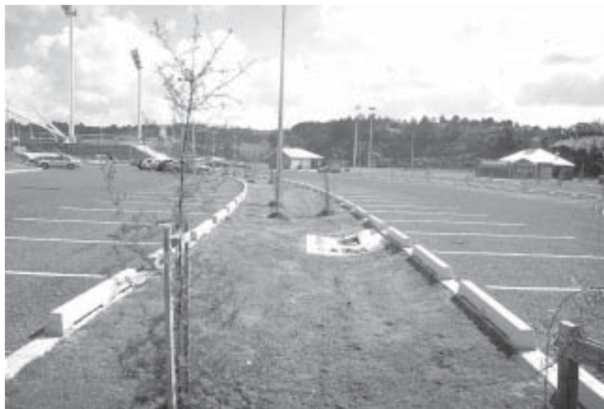
Biofiltration Swale at the North Harbour Stadium
