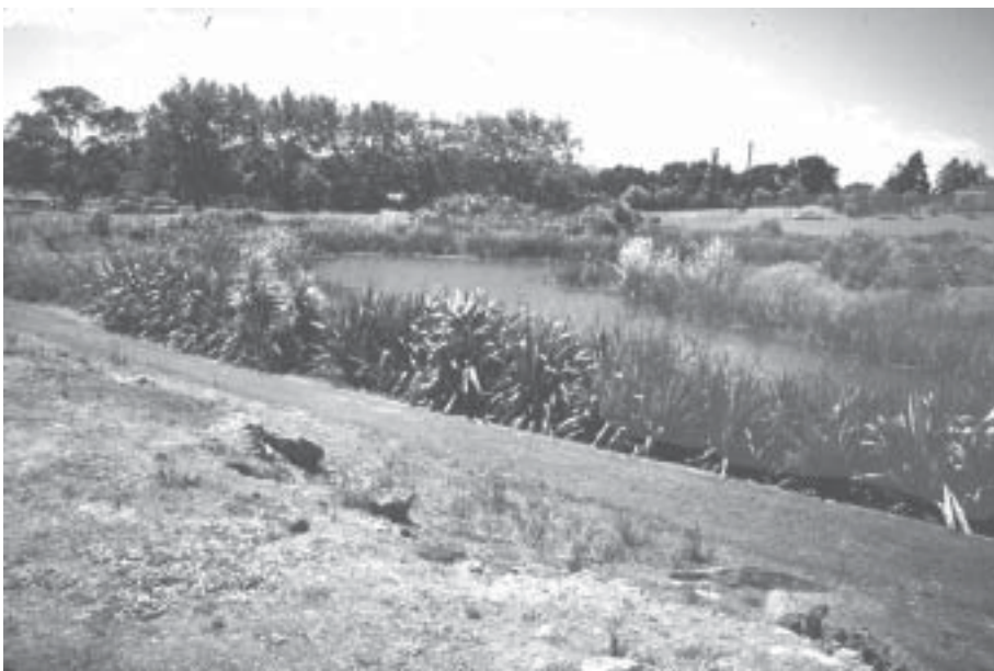
Stormwater Wetland Fringe Pond Used for Water Quality Treatment
