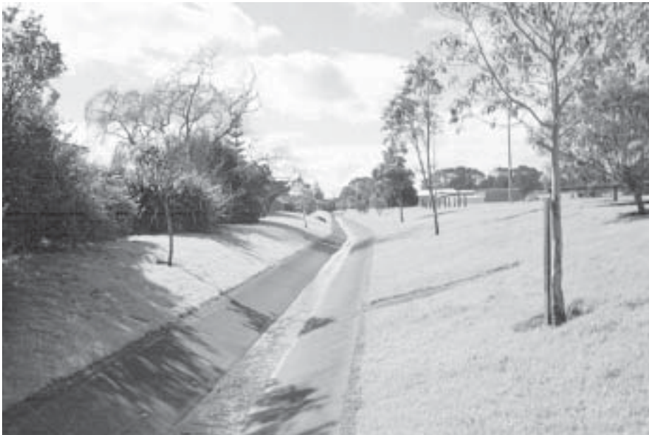
An Efficient Stormwater Conveyance System. Rapid Travel Through the System Precludes any Water Quality Treatment
