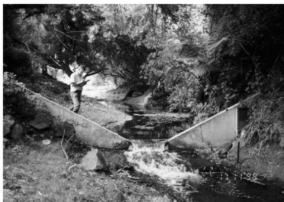
Plate 8: Flow measuring weir on Meola Creek.
