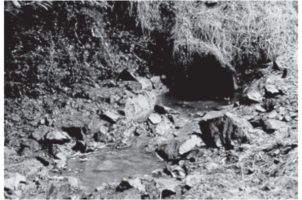
Plate 15: Series of rock weirs built to drown culvert outlet.
