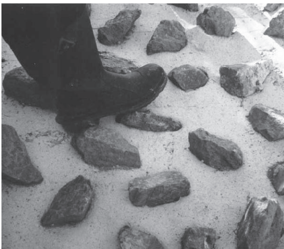
Plate 17: An example showing how rocks could be used to increase the channel roughness of a culvert.
