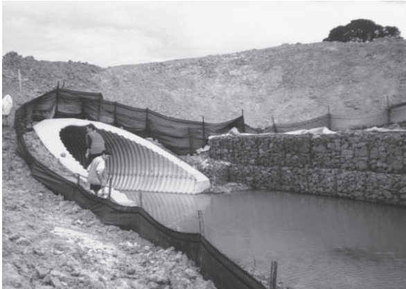
Plate 16: Erosion control at culvert outlet.
