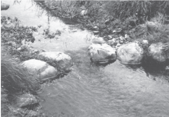
Plate 19: Notched weir constructed from large rocks.
