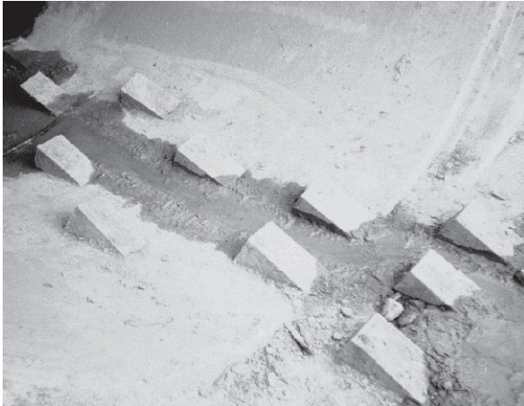
Plate 18: Spoiler design installed in an Auckland culvert.
