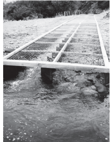
Plate 20: Combined Denil and nature-like fishway installed to allow passage of trout and indigenous fish species. The netting on top was included to prevent predation by birds.
