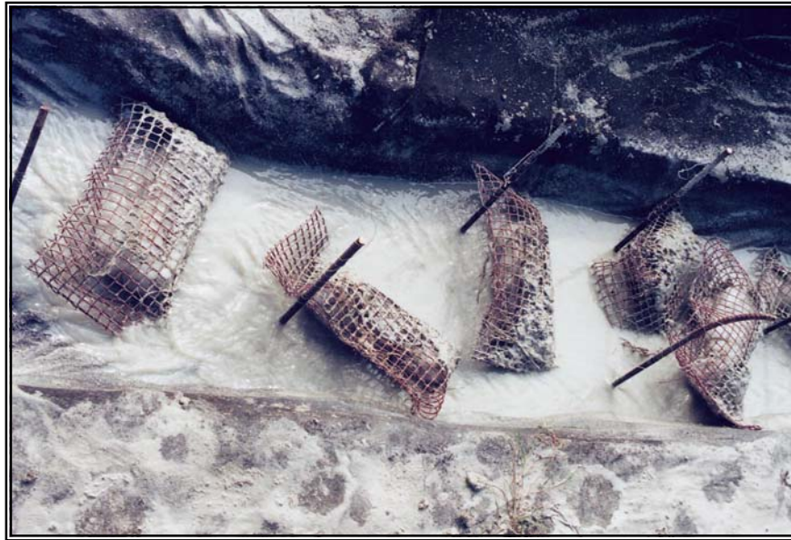
Figure 9: Floc Blocks within Channel between Forebay and Pond
