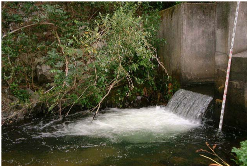
Figure 4: Water gauging flume located on the Mangatangi Stream, approximately 2 kilometres downstream of the Mangatangi Dam.
