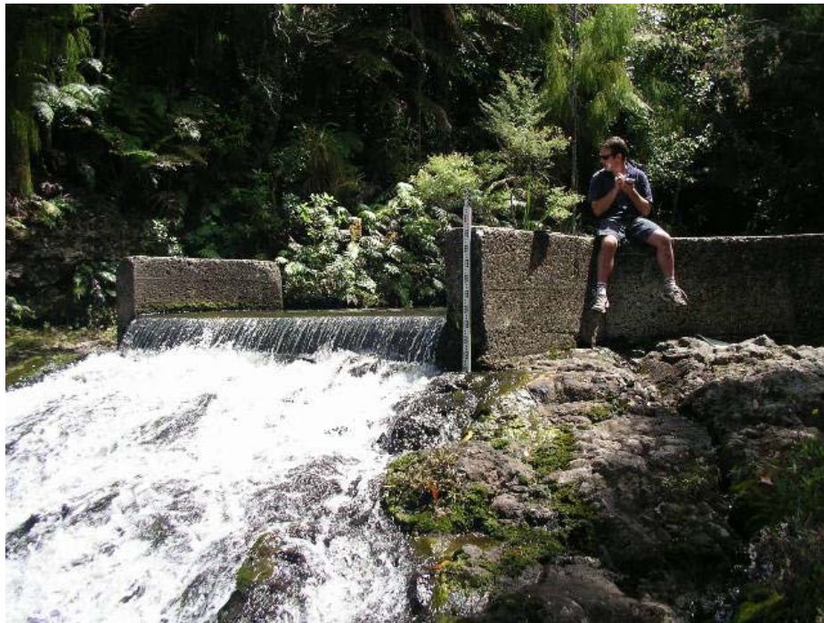
Figure 4: Watercare Services Ltd water gauging flume located on the Nihotupu Stream, approximately 200 m upstream of the Upper Nihotupu Reservoir.
