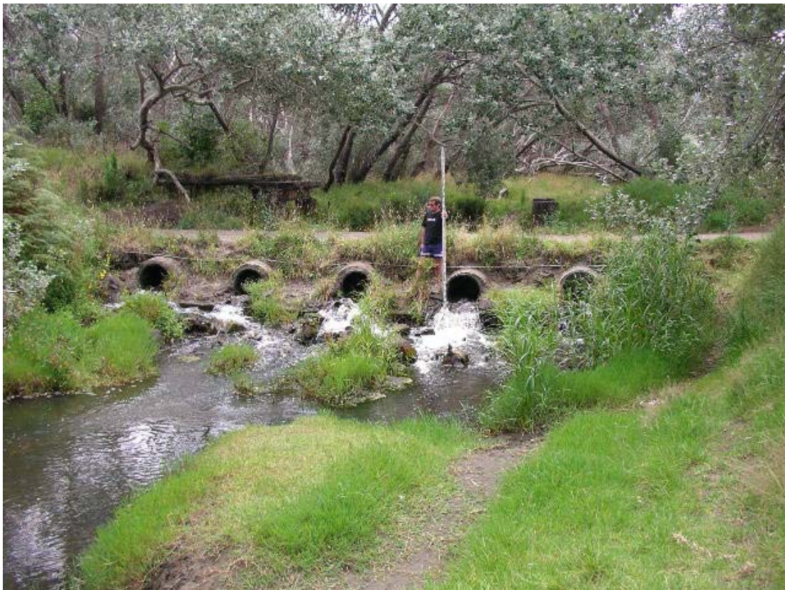
Figure 6: Five barrel ford located on the Okiritoto Stream within the Muriwai Regional Park
