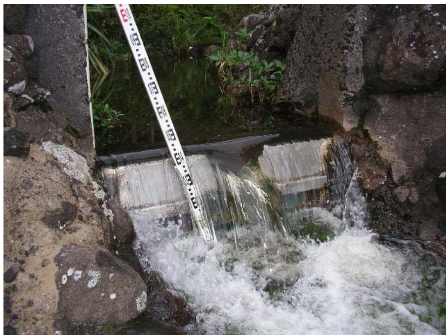
Figure 5: Obsolete water flow-gauging weir located on the Waitakere River above the Waitakere falls, but below the dam.
