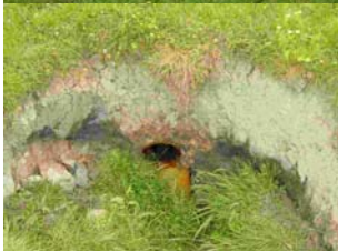
WS1 C, showing catchment and a collapsed tile drain (also found at site A and B).
