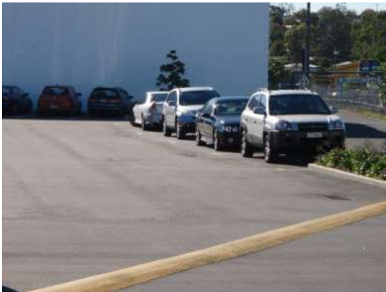
Figure 55 Mitre 10 Mega ponding area: water is contained in the low point by the kerb and speed hump
