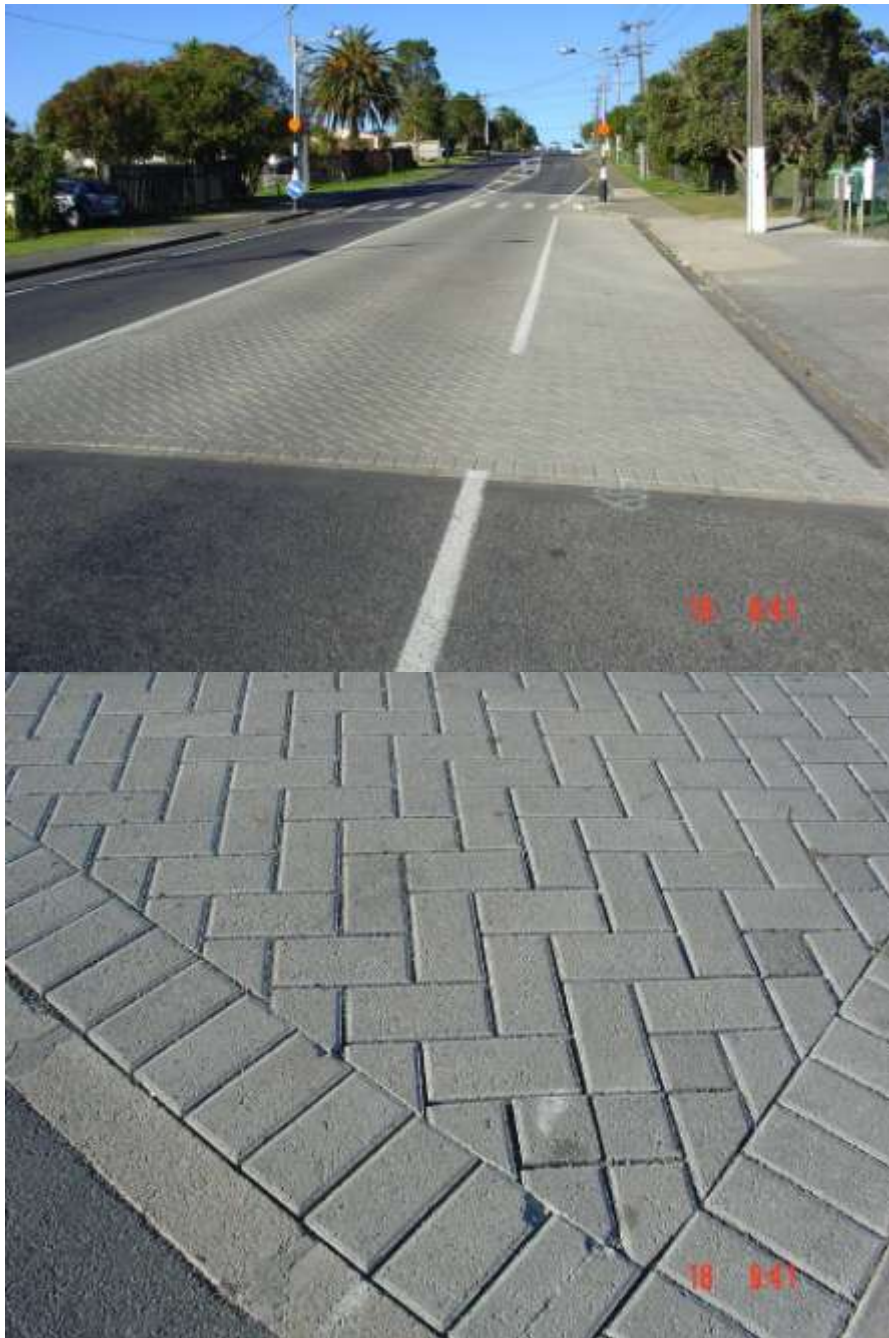
Figure 27 Birkdale Rd permeable paving (Timperley M. 2008)
