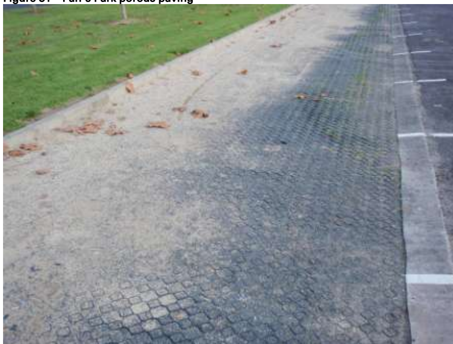
Figure 31 Parr's Park porous paving
