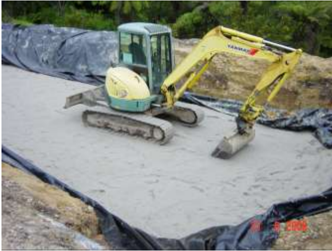
Figure 39 Paul Matthews rain garden under construction: placement of sand (Boffa Miskell 2008)
