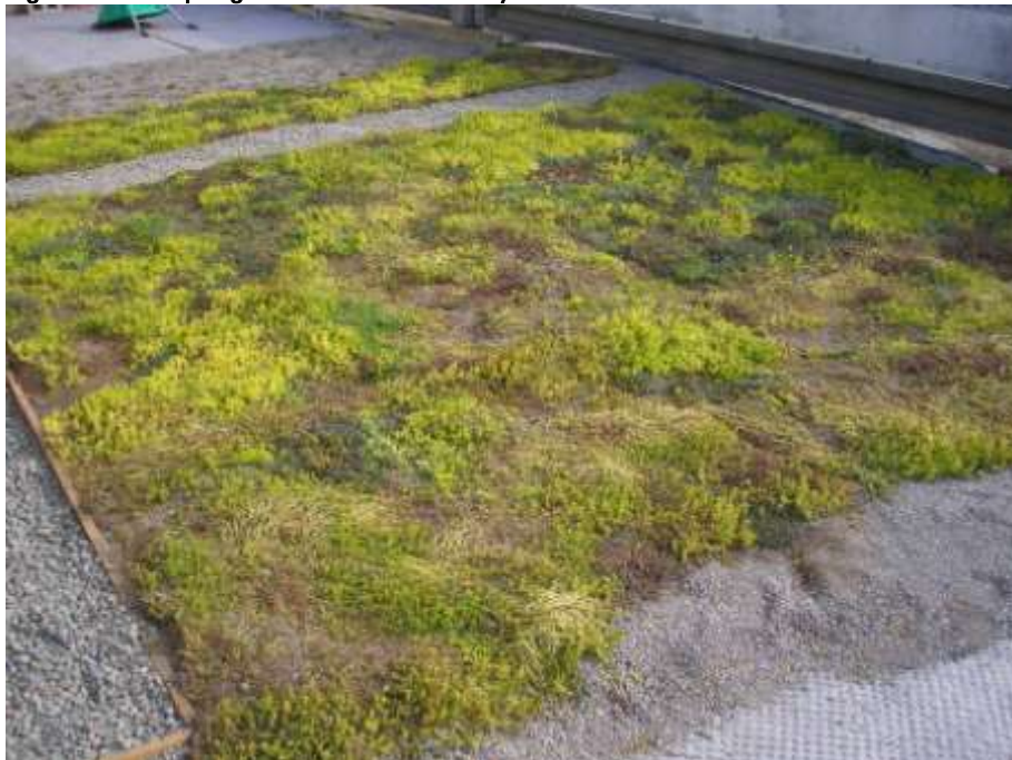
Figure 24 The pre-grown mats immediately after construction
