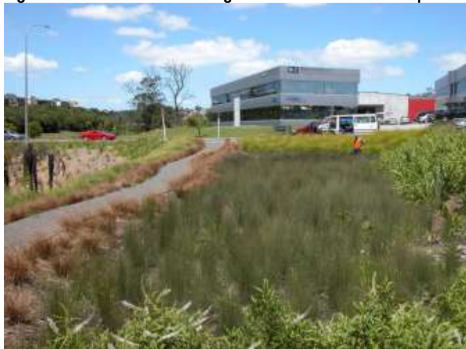
Figure 40 Paul Matthews rain garden under construction: placement of sand (Boffa Miskell 2008)
