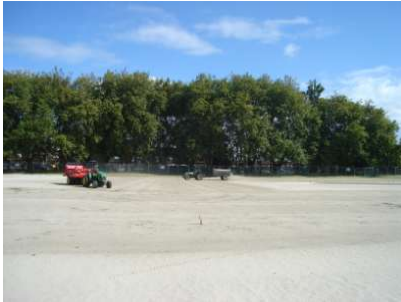
Figure 20 An application of a sand followed gravel banding to protect the top of the bands during field use. The turf grass grew through the sand layer to stabilise it (after SSDM, 2009).
