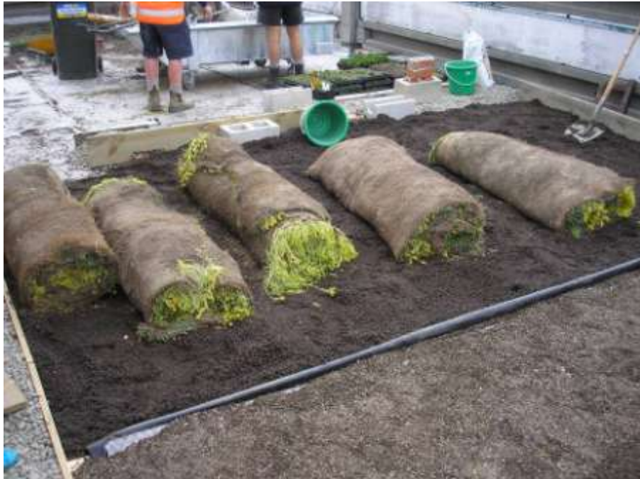
Figure 23 These plots were planted with pre-grown mats to improve plant density and establishment
