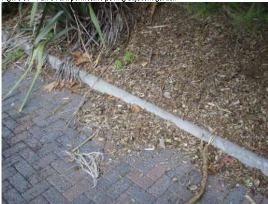
Figure 30 Parr's Park permeable paving adjacent garden
