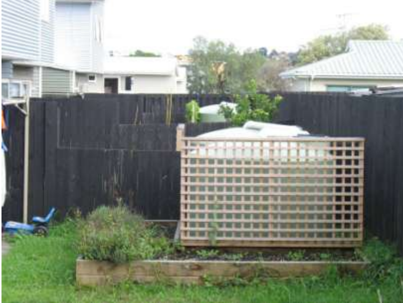
Figure 46 Talbot Park: rain tanks for three bedroom houses
