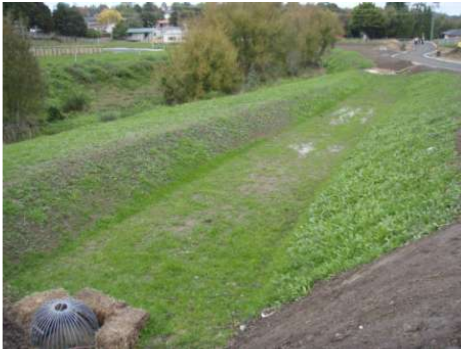
Figure 43 New Zealand Housing Foundation, Albionvale: swale prior to planting
