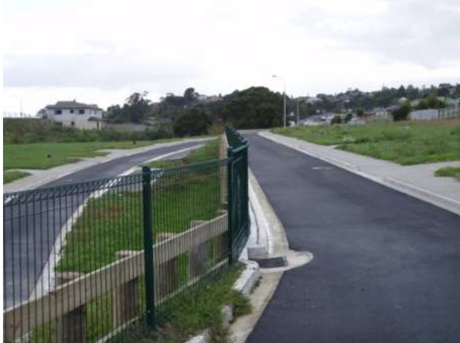
Figure 17 New Zealand Housing Foundation: subdivision layout with narrow roads and parking bays
