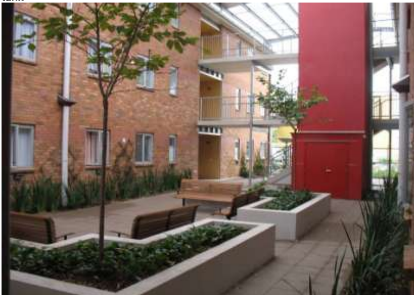
Figure 47 The Atrium courtyard: large downpipes on the walls direct roof water to the underground tank
