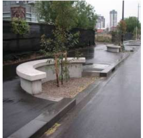
Figure 33 Other Dockland tree-pit examples with inflow directly from the street surface and through a grate. Notice the use of a seating wall to avoid conflicts with pedestrians (right) (Haycox, M. 2005)
