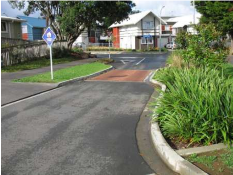
Figure 18 Talbot Park: road widths change at the entry points to the development
