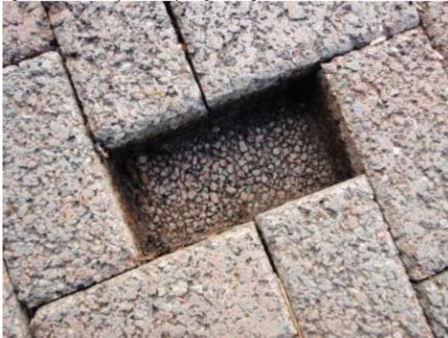
Figure 29 Parr's Park permeable paving showing basecourse
