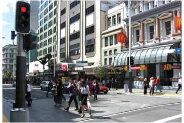
A newly created mid-block street crossing, Queen Street.
